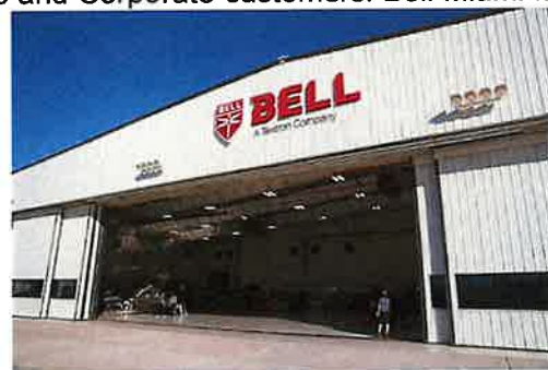
Figure 1-11. Bell Miami Service Center.
