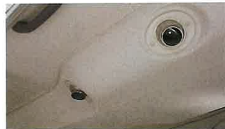
Figure 2-14. Headliner with Air Conditioning Ducting.
