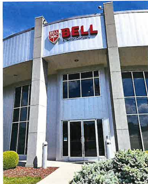
Figure 1-14. Bell Piney Flats Service Center.
