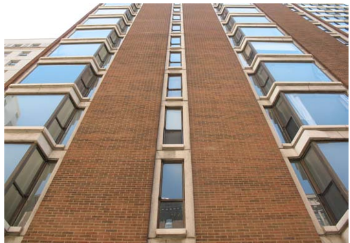
Vertical bands of brick alternating with projecting bays gives the building a striped appearance
