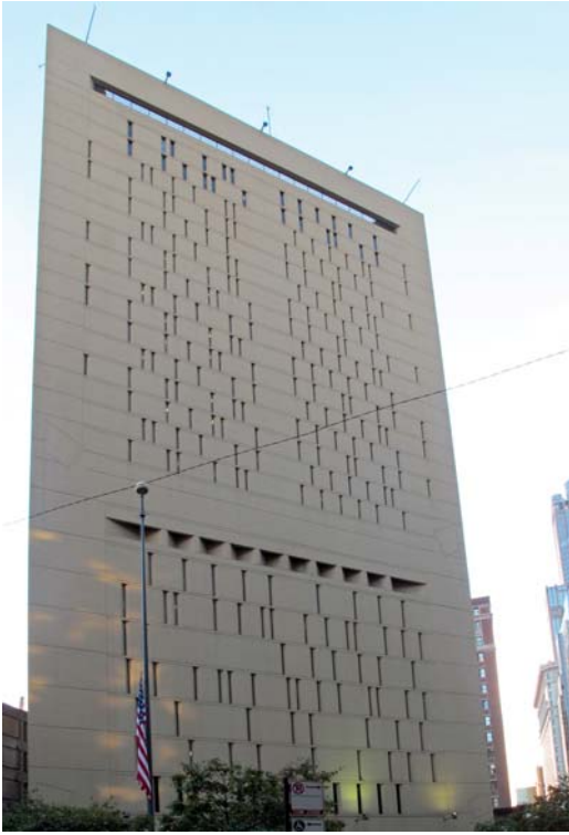
Oak Park Village Hall, 123 Madison Street (1975)
