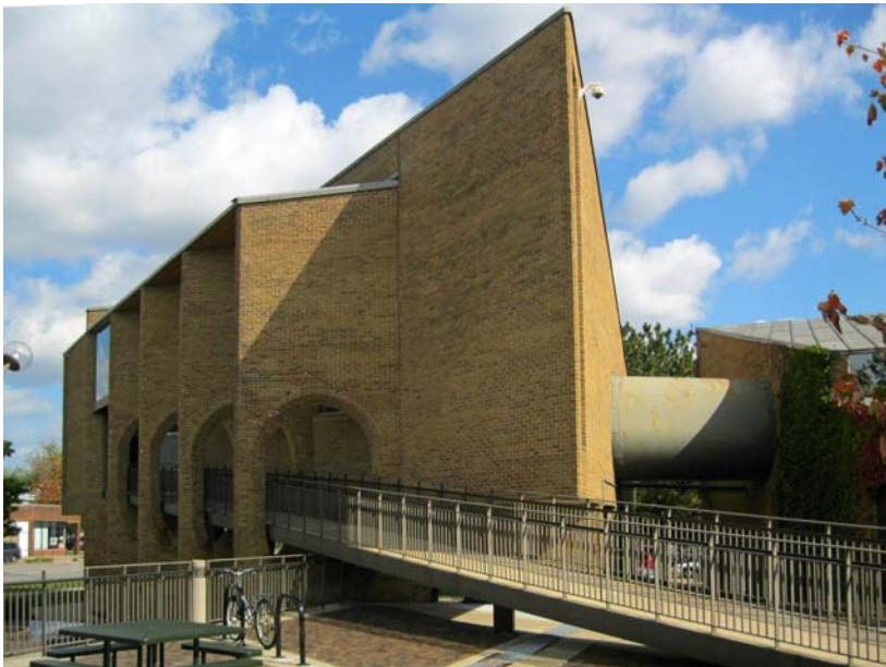
Time-Life Building, 541 N. Fairbanks Court (1968)
