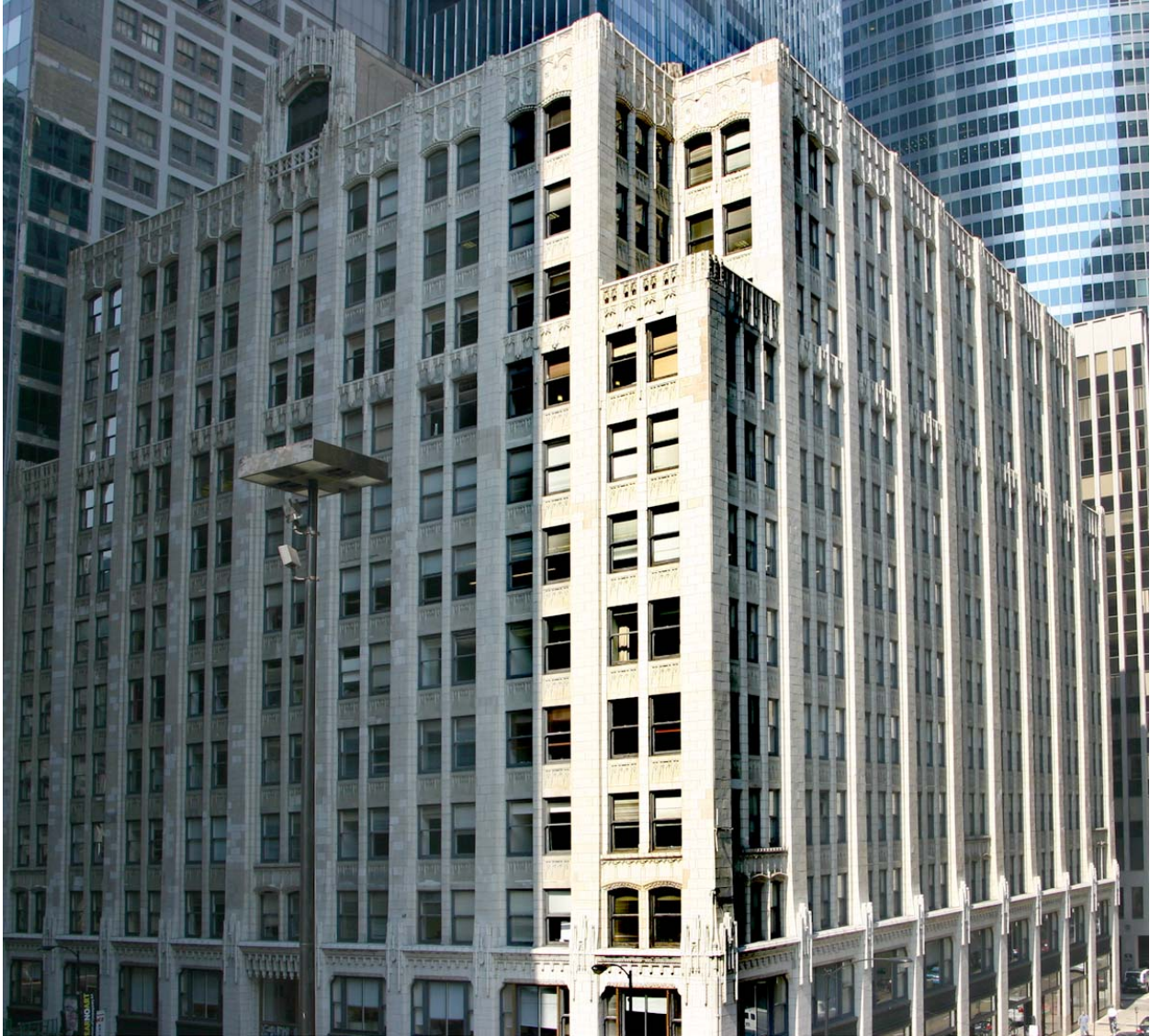
The building is a 12-story terra cotta-clad office building built in the Gothic Revival style.
