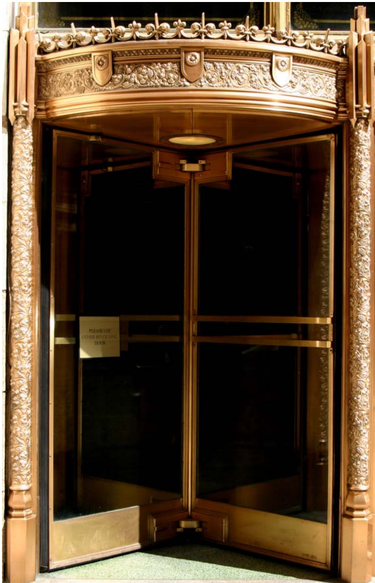
One of the building's elaborately-detailed entrance doors.
