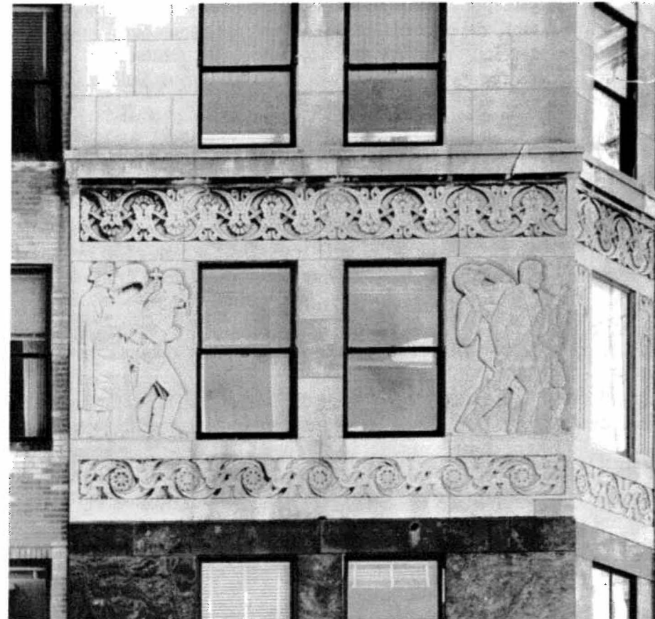
The 333 North Michigan Building includes a fifth-story frieze relating to Chicago's early pioneer life, as befitting a building located on the former site of Fort Dearborn. Among the images that were depicted by sculptor Fred M. Torrey (clockwise, from upper left): "The Hunter," "The Indian," "The Pioneer Woman," "The Struggle," and "The Missionaries."
