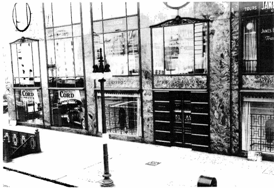
Cast-iron storefronts line the base of the 333 North Michigan Building, which is sheathed in polished granite in variegated shades of black, purple, gray, and pink. The building has changed little from its appearance at the time of this mid-1930s photograph, although the Duesenberg auto dealership (lower left) vanished long ago. The building's elongated floor plan (top) still provides a variety of retail and office arrangements.
