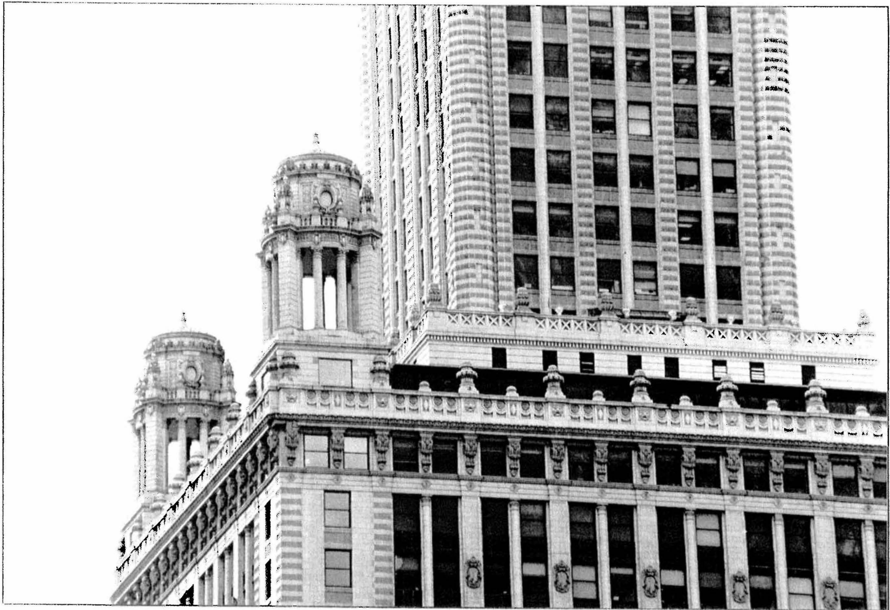
View of the upper stories of the building and of the set-back at the base of the tower. The pavilions at the corners originally concealed water towers used as a source for the sprinkler system. The only significant alteration to the building is visible here behind the parapet at the 24th floor; a steel and glass enclosed extension of the renovated spaces that formerly housed mechanical systems. (Photograph by Timothy N. Wittman for the Commission on Chicago Landmarks)
