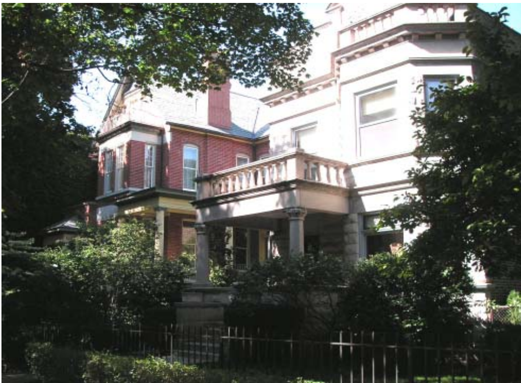
Top and above: The District is a mix of free-standing houses, row houses, apartment buildings, and institutional buildings predominantly from the late nineteenth and early twentieth centuries.
