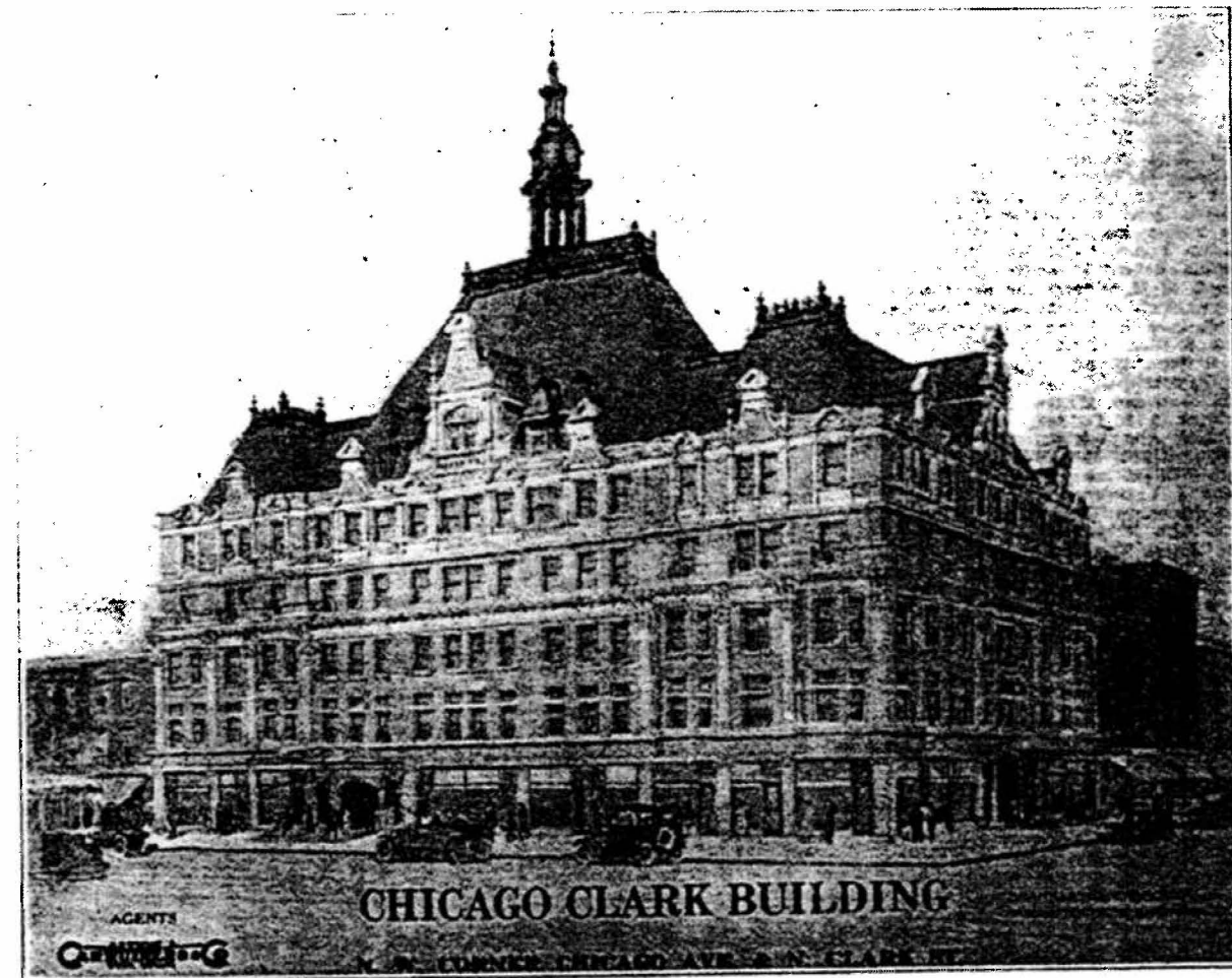
THE CHICAGO CLARK BUILDING 800-810 NORTH CLARK STREET AND 100-112 WEST CHICAGO AVENUE
