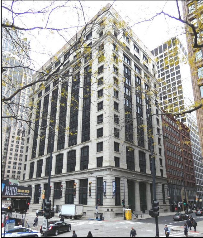
The south and west façades are clad with a light-grey granite ( top left ), and the rear with cream-toned brick ( top right ).
