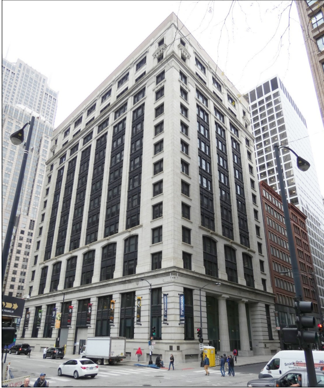
Main south and west elevations of the Chicago & North Western Railway Office Building. The granite-clad fourteen-story building was completed in 1905 and designed by the Chicago firm of Frost and Granger.
