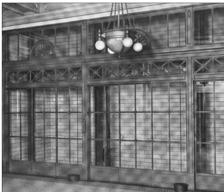
Left: Windows throughout the building feature cast-iron mullions and spandrel panels with geometric ornamentation created by the Winslow Brothers Company, one of Chicago's leading manufacturers of decorative metalwork. The Winslow Brothers also created cast-iron interior features for the building such as the lobby elevator doors in this circa 1905 photo from the Winslow Brothers company 1910 catalog.
