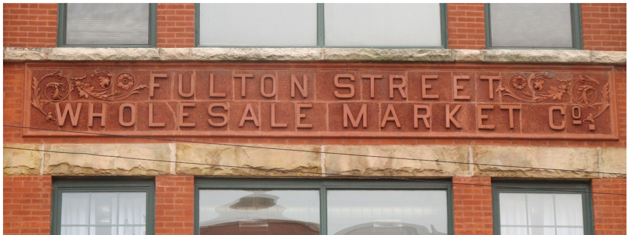
The south of two rows of meat packing buildings built in 1887 by a consortium of meat packing firms. By at least 1902, the “big three” meat packing firms in Chicago and the nation—Philip Armour, Gustavus Swift and Nelson Morris—all had branch operations in this complex and its counterpart structure across the street.
