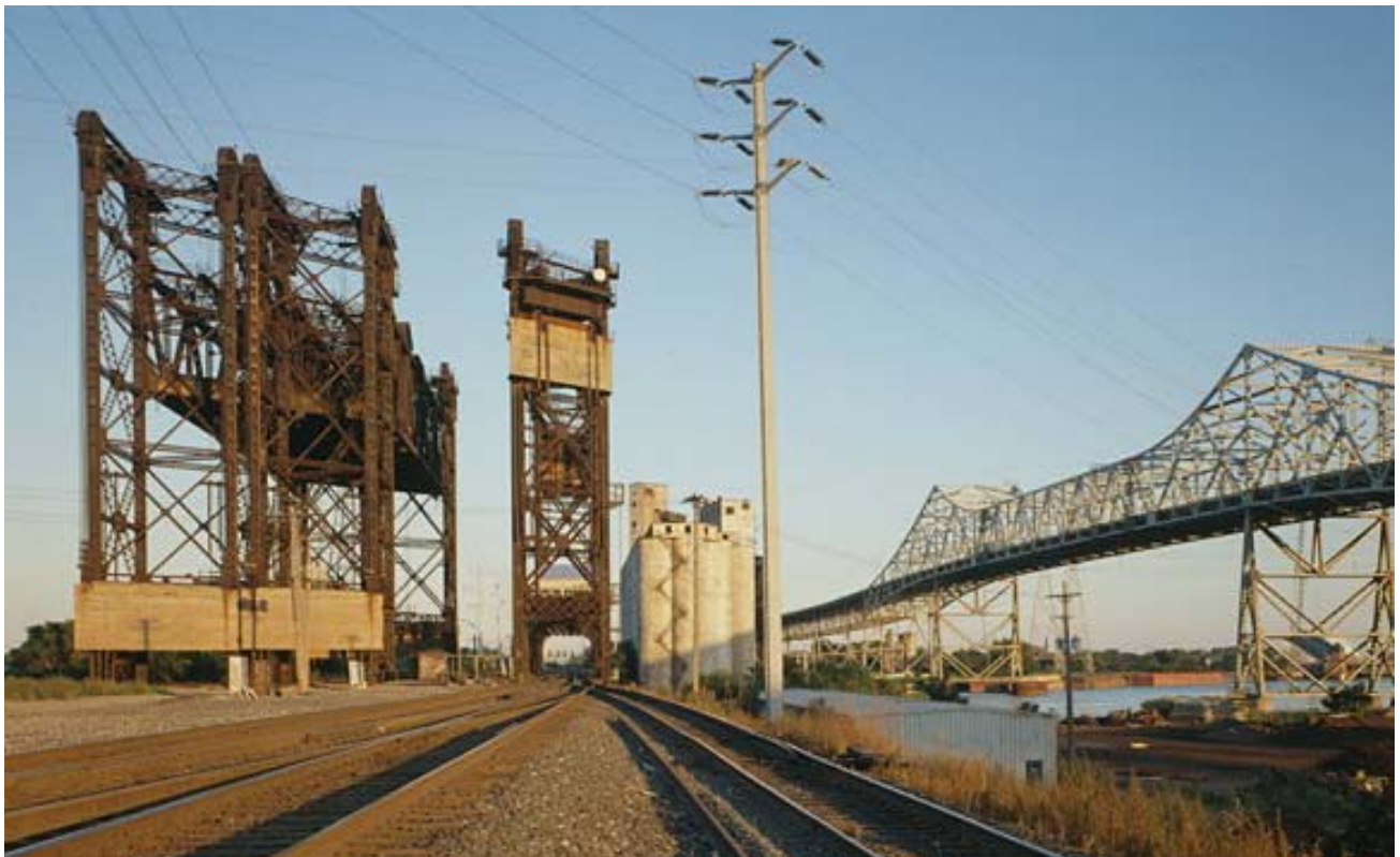
Top: The Lake Shore & Michigan Southern Railway Bridges are two adjacent, double track, steel-truss spans that together make up the largest multiple installation of Waddell and Harrington vertical-lift bridges. Bottom: Situated immediately west of the LS&MS pair of bridges is a portion of a span that once was part of the Pittsburgh, Fort Wayne & Chicago Railway Bridge (center) and further west is the Chicago Skyway (far right).
