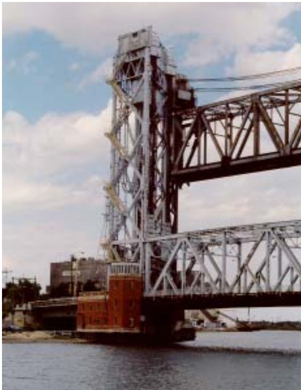
Top: The Chicago & Western Indiana Railroad Bridge is an outstanding example of a “tower-driven” vertical-lift bridge. Left: The span was designed to be raised and lowered by a system of giant pulleys and cables.
