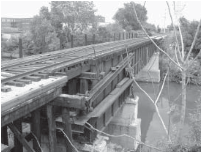
The Chicago & Illinois Western Railway Bridge is a rare-surviving example of a bridge design by Theodor Rall, a leading railroad bridge engineer. The bridge features a single leaf attached to a main roller (above). Near the bridge's counterweight are struts and a trunnion (left) that, when engaged, raise the leaf.
