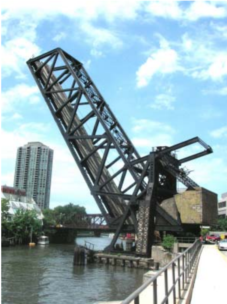
Left: The Chicago & Northwestern Railway Bridge on the North Branch of the Chicago River is an excellent early example of an overhead-counterweight bascule bridge based on the patents of prominent Chicago bridge designer Joseph Strauss. Bottom: The bridge's massive concrete counterweight weights over 1,200 tons.
