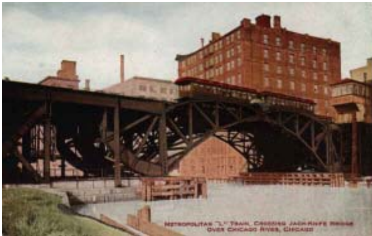
William Scherzer's rolling lift bridge at Van Buren St. (left) represented an unparalleled advance in the design of moveable bridges. The design of other bascule bridges, based on the principals of Scherzer's design, included the Strauss Bascule Bridge by Joseph Strauss (bottom left). Strauss' bridge for the Chicago & Northwestern Railway (listed as Bridge 6 in this report) is seen below in 1908.
