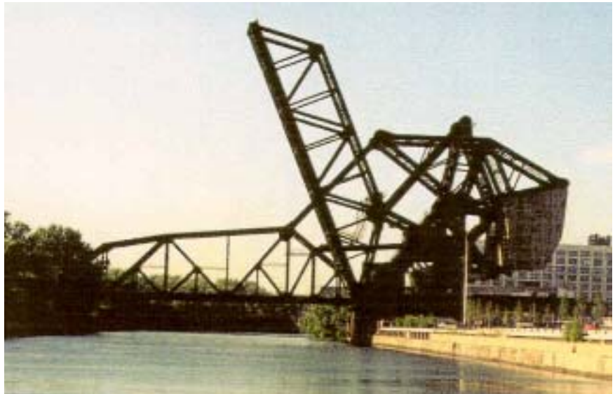
The SCAL Bridge (above) was the world's longest and heaviest bridge upon its completion in 1919. The bridge was shortened and moved to its current location in 1930 following the straightening of the South Branch of the Chicago River.
