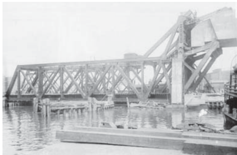
William Scherzer's rolling lift bridge at Van Buren St. (left) represented an unparalleled advance in the design of moveable bridges. The design of other bascule bridges, based on the principals of Scherzer's design, included the Strauss Bascule Bridge by Joseph Strauss (bottom left). Strauss' bridge for the Chicago & Northwestern Railway (listed as Bridge 6 in this report) is seen below in 1908.
