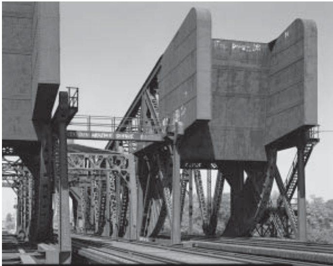
The Pennsylvania Railroad “Eight-Track” Bridge is significant for being the last Scherzer Rolling-Lift Bridge erected in Chicago for railroad use. The bridge encompasses four side-by-side bridges (bottom right). The counterweights are situated on alternating ends of each span (bottom left).
