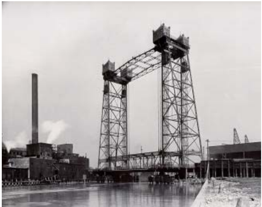
During the late-1890s, Chicago emerged as the nation's center for the study of moveable bridge design. Two important moveable bridge types introduced in Chicago were the rolling bascule bridge at Van Buren St. designed by William Scherzer (middle) and the vertical-lift bridge at Halsted St. developed by J.A.L. Waddell (bottom).
