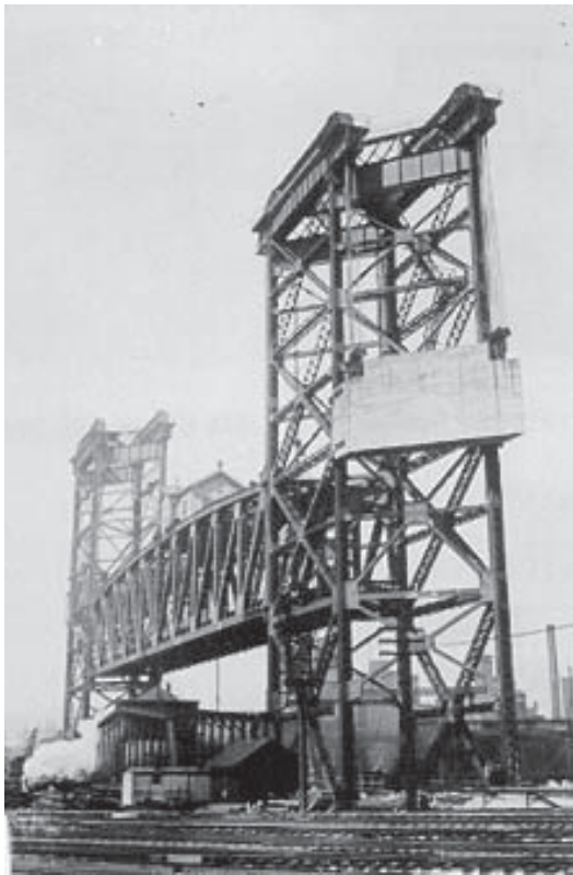
The design and construction of innovative bridges in Chicago by prominent designers put Chicago on the cutting edge of moveable bridge design. J.A.L. Waddell (top center) and John Harrington (top right) collaborated to design acclaimed vertical-lift bridges. One of their designs, the Pennsylvania Railroad Bridge (listed at Bridge 4 in this report) is shown in the late 1910s (left).
