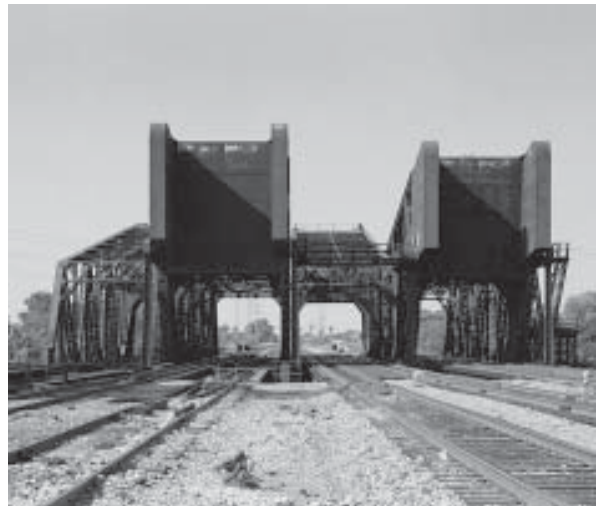
The Pennsylvania Railroad “Eight-Track” Bridge is significant for being the last Scherzer Rolling-Lift Bridge erected in Chicago for railroad use. The bridge encompasses four side-by-side bridges (bottom right). The counterweights are situated on alternating ends of each span (bottom left).
