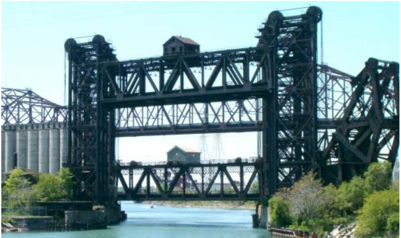
Top: The Lake Shore & Michigan Southern Railway Bridges are two adjacent, double track, steel-truss spans that together make up the largest multiple installation of Waddell and Harrington vertical-lift bridges. Bottom: Situated immediately west of the LS&MS pair of bridges is a portion of a span that once was part of the Pittsburgh, Fort Wayne & Chicago Railway Bridge (center) and further west is the Chicago Skyway (far right).
