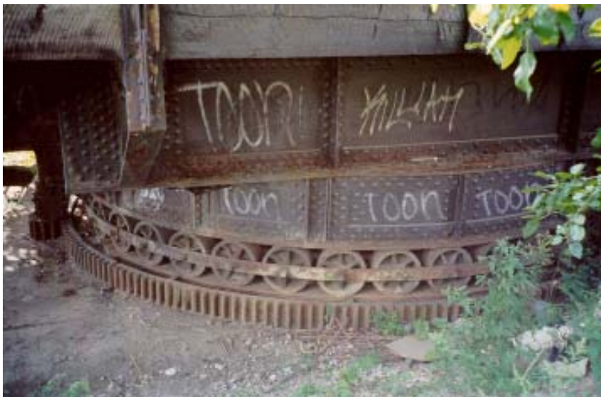
The Chicago, Milwaukee & St. Paul Railway Bridge is a rare asymmetrical bobtail-swing bridge. It rests on a pivot pier (above left) on the north embankment while the span stretches across the North Branch of the Chicago River (above right).
