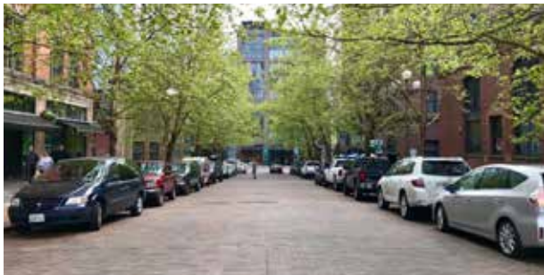
Examples of using pavers for traffic-calming
