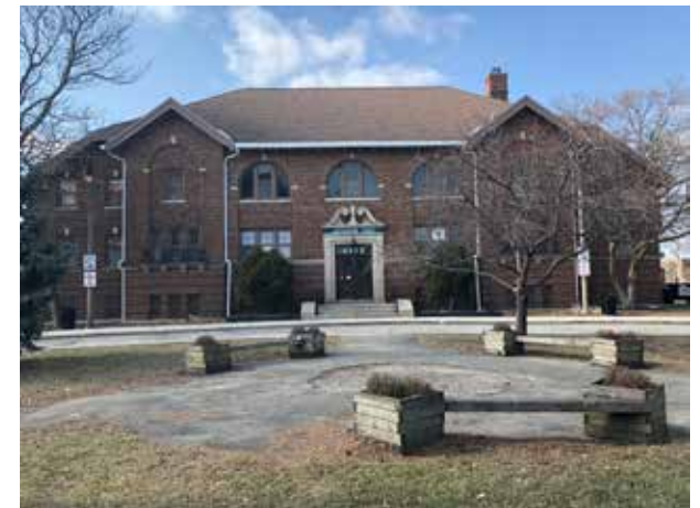
The Jefferson Park Fieldhouse is an important destination for the community. Property maintenance is critical to a sense of safety and comfort.
