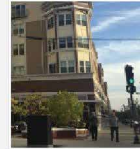
A building setback above the building base frames the street and establishes a comfortable pedestrian experience
