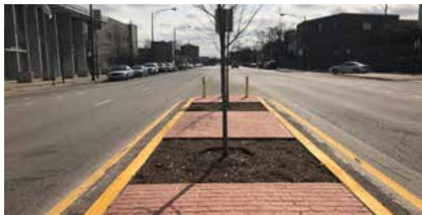
New pedestrian island installed on Milwaukee near Foster Ave.
