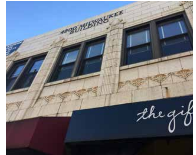
Windows should be grouped and be proportional to the building to help establish rhythms across a facade.
