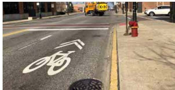
New shared lane markings
