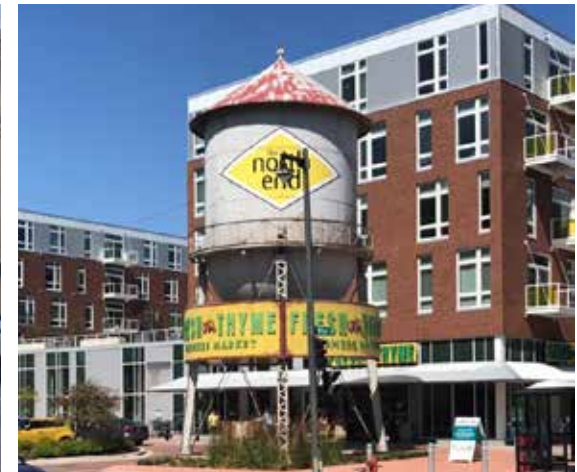
This example illustrates the type of mixed-use development that provides a number of amenities and a pedestrian-oriented environment. (Milwaukee, WI)
