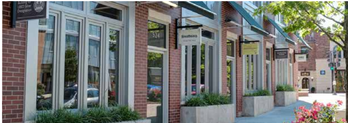
Examples of live-work spaces in Logan Square, Chicago and in Evanston, Illinois
