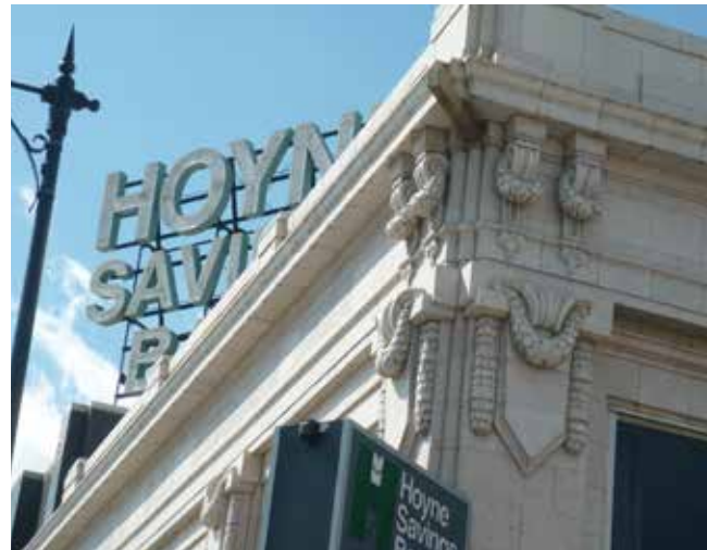
Jefferson Park is home to many iconic older buildings, like the Hoyme Bank building at Milwaukee and Lawrence, and these should be preserved and enhanced.
