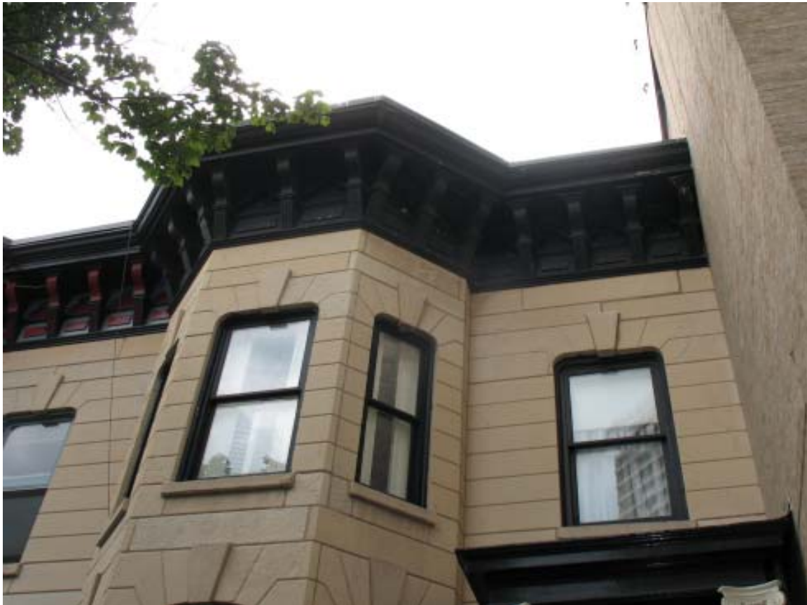
The Lincoln Avenue Row House District's buildings were designed in the Italianate architectural style, popular in Chicago in the 1860s through 1880s.
