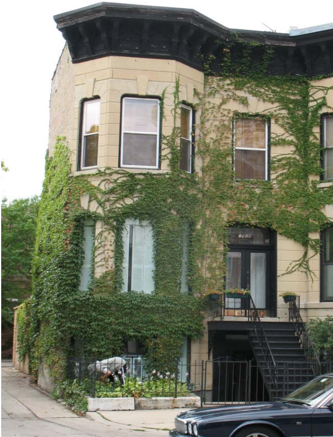
A view of 1928 N. Lincoln Ave. Each row house in the Lincoln Avenue Row House District is faced with large blocks of Joliet limestone.
