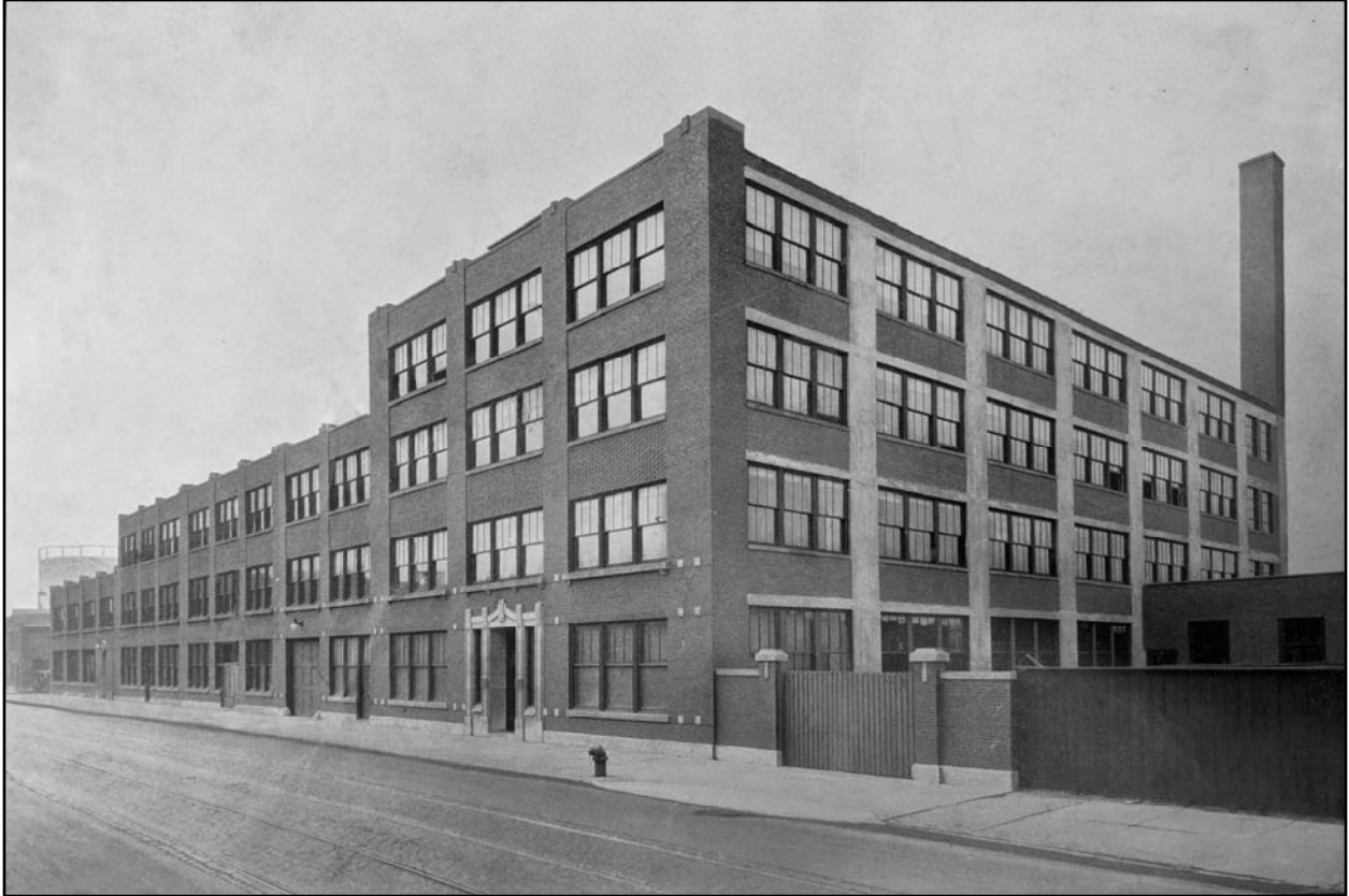
Above: Looking south along Clybourn Avenue circa 1928, showing Blocks 1 through 4 of the Ludlow Typograph Company Building. The same view is shown below in 2021.
