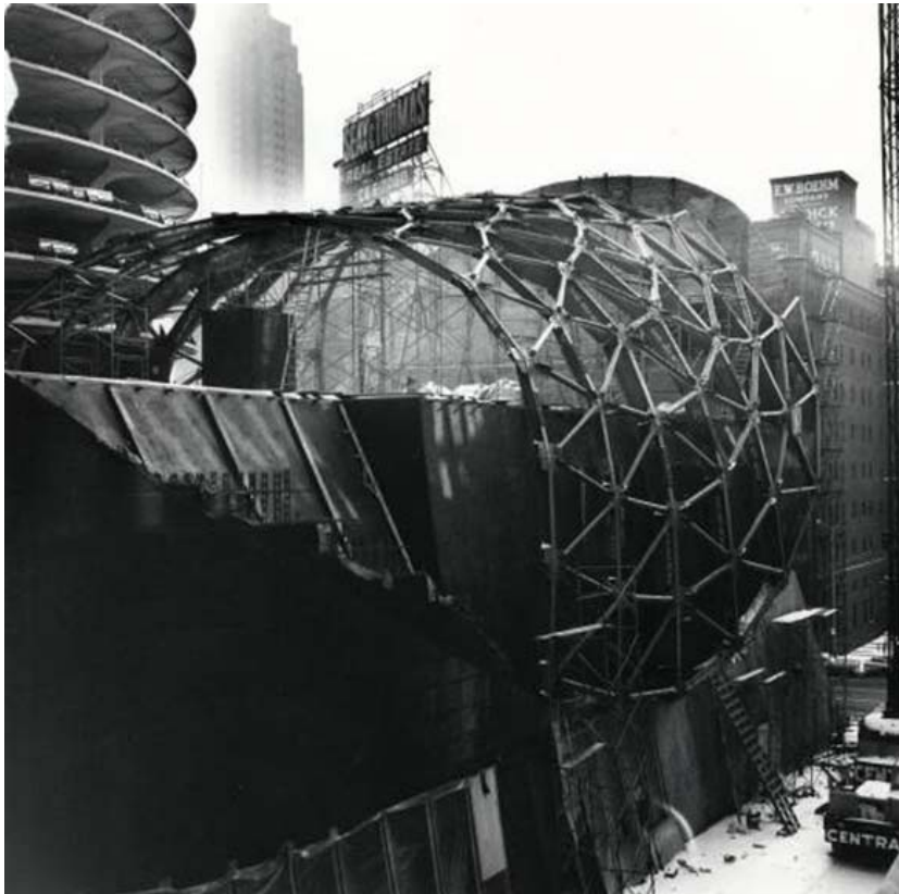
Construction on the office building (above, photo by Bertrand Goldberg Associates, October 1962) and the theater building (left, ca. 1966, from Ragon's Goldberg, Dans La Ville / In the City ) continued through the mid-1960s, with the saddle-shaped theater, the last element in the complex, completed in 1967.
