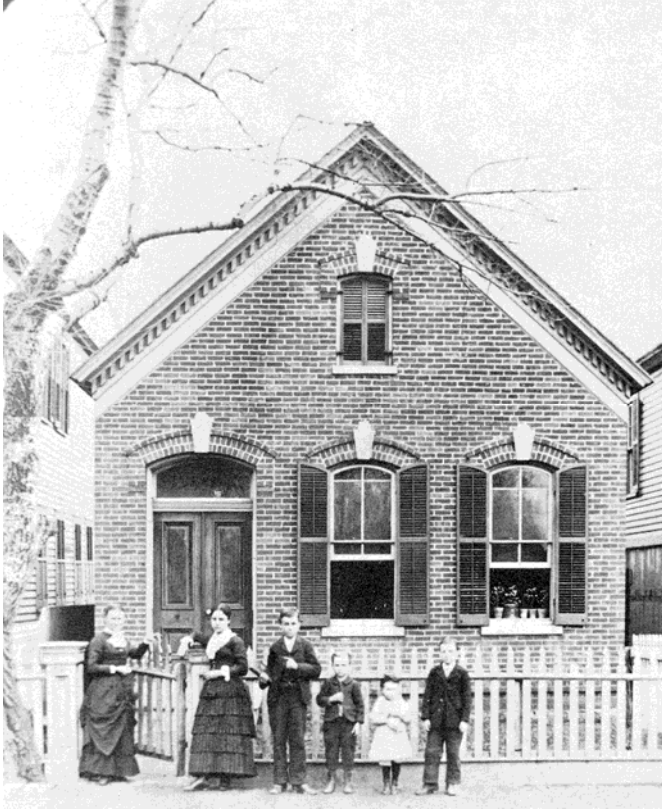
Later cottages, especially those built after the 1871 Chicago Fire, were built of brick. Top: A simple Italianate-style cottage with stone keystones set within arched brick lintels.
