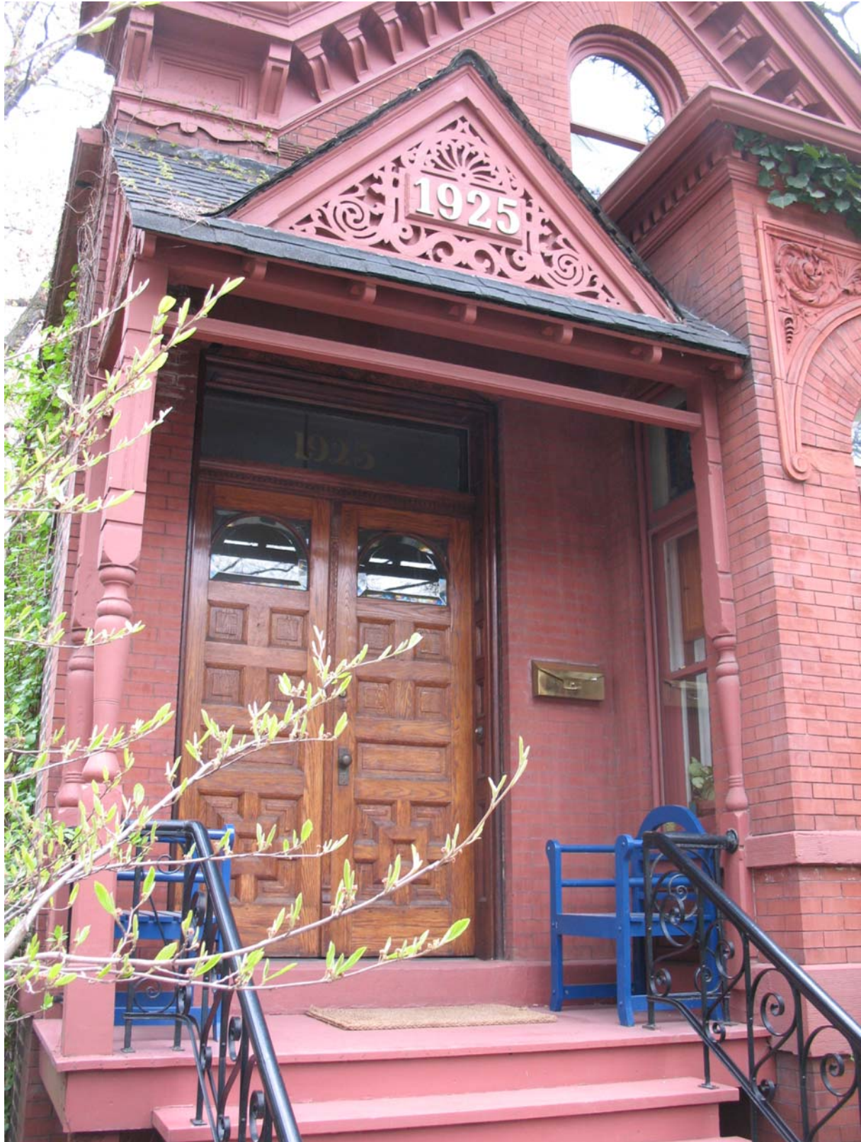
The Schnitzius Cottage's front porch combines turned-spindle posts with jigsaw-cut curvilinear ornament. The building's pair of front doors are finely paneled in wood.
