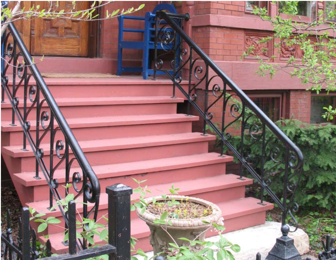
Details of the front porch's wood roof and cast- and wrought-iron railings.
