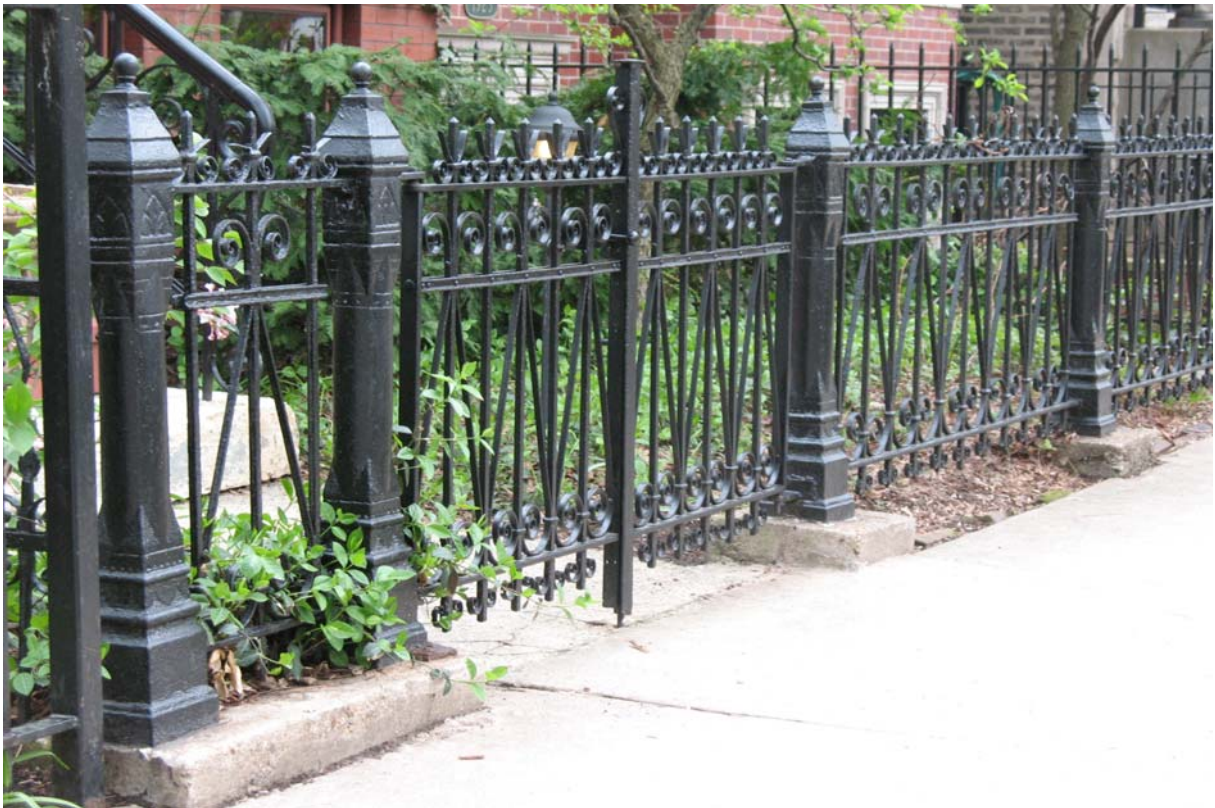
The Schnitzius Cottage retains all of its decorative-metal exterior detailing, highly unusual in the context of nineteenth-century Chicago residential buildings. Top: A view of the building's pressed-metal cornice, ornamented with brackets and dentils. Bottom: The building's cast- and wrought-iron front fence.
