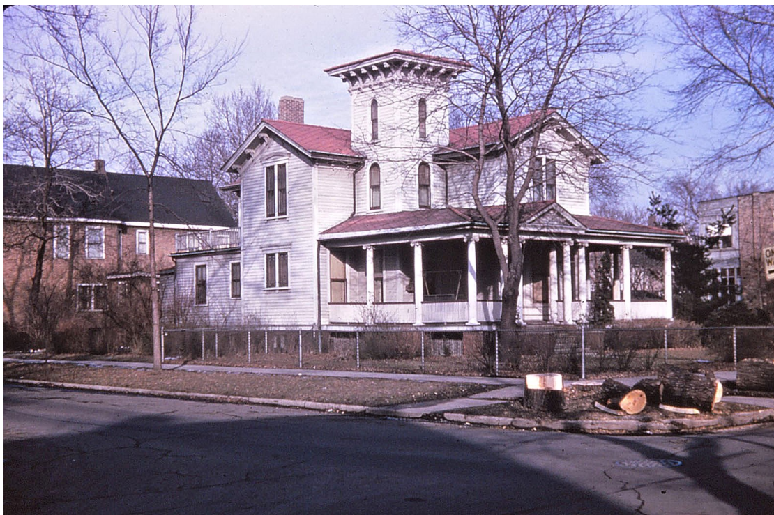
The Gray House, as captured in 2023 (Above) and in a 1950s photo, a century after its initial construction (Below). Based on historic maps, and the presence of both the wraparound front porch and the one-story rear wing, this is how the farmhouse appeared from ca.1924 through the late 1980s. Source: Troy Walsh, Drone Media Chicago (2023); Kris and David Cloud
