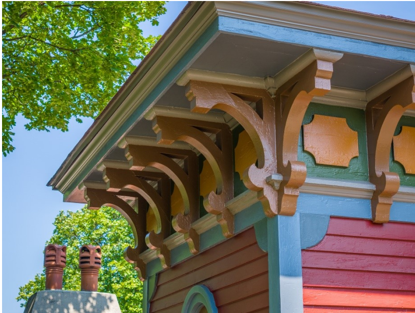
Left: Bracketed cornice and decorative frieze band under the eaves of the tower's hip roof.
