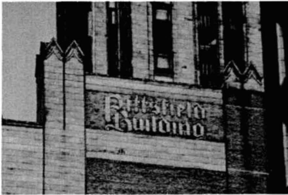
Top and bottom: The upper floors of the Pittsfield Building are clad with gray terra cotta in a variety of ornament, both geometric and foliate, that combines both Gothic and Art Deco influences.
