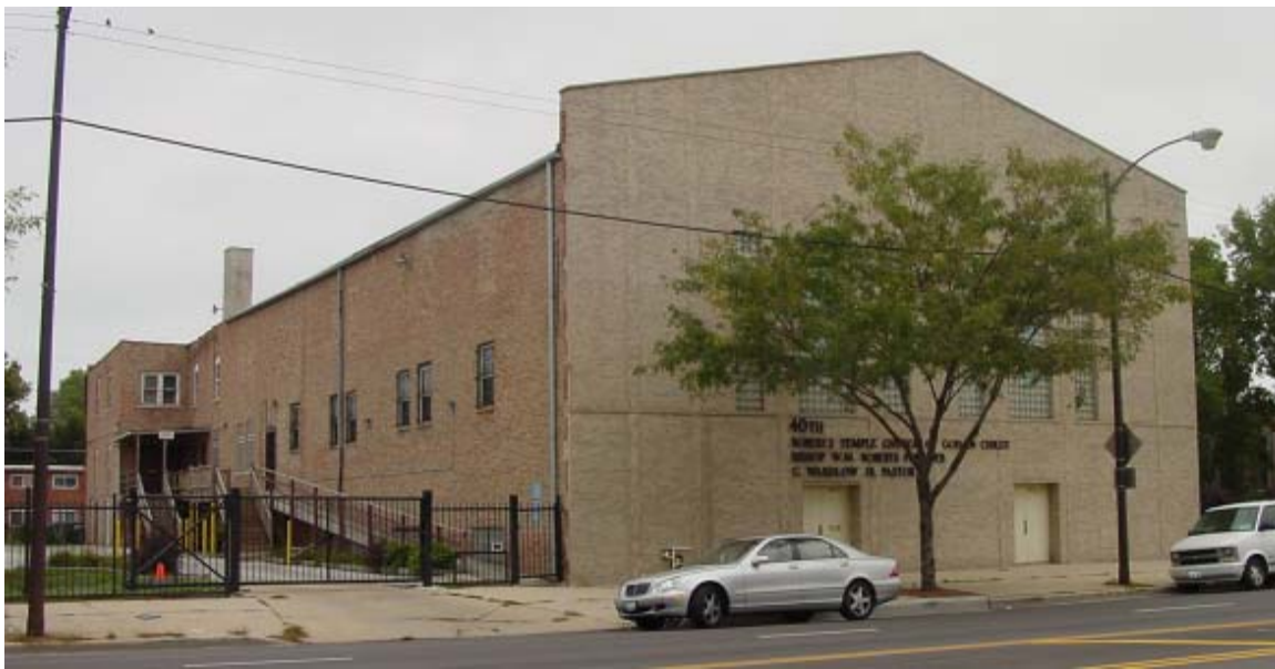
Views of the Roberts Temple Church of God in Christ Building as of October 2005. Although the front facade of the building was covered with new brick in 1992-93, the historic red brick of the front facade remains behind it. The original massing, roof form, and other elevations all remain.
