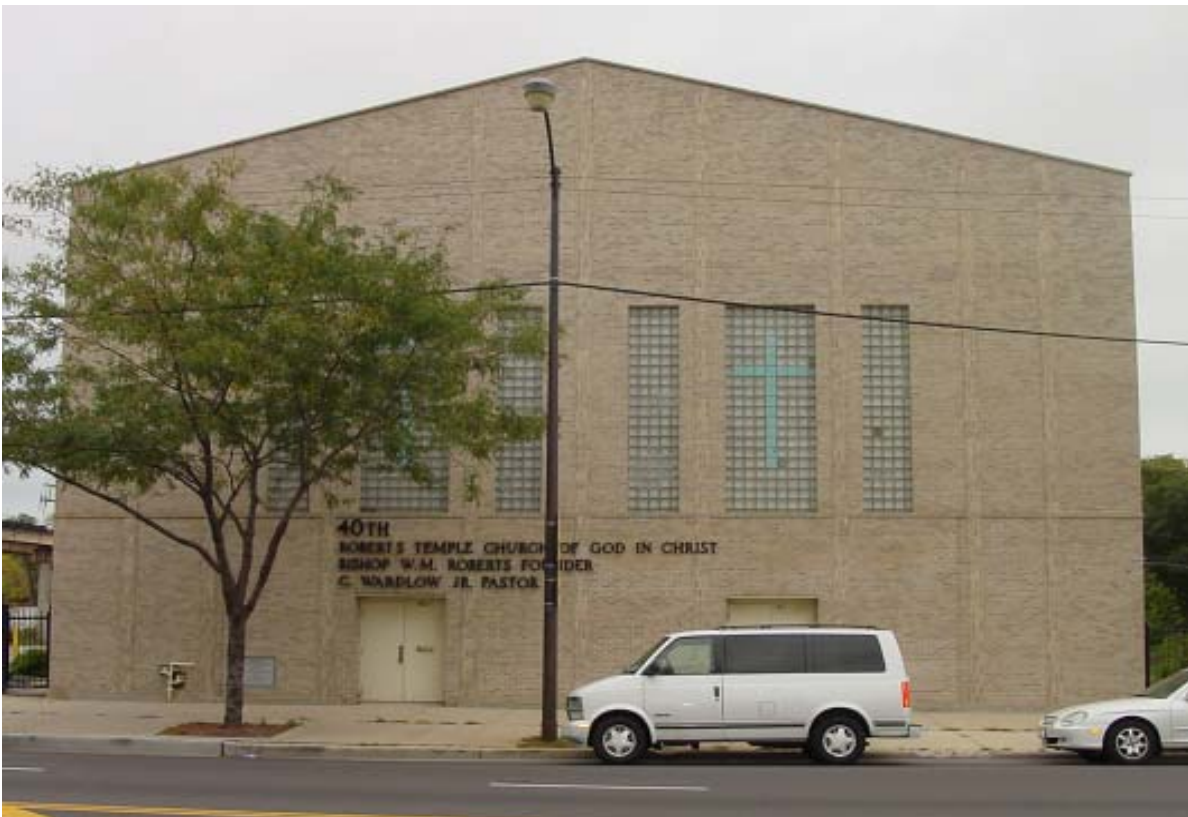
Top: A historic view of the Roberts Temple Church of God in Christ Building much as it appeared in 1955 (photographs of the Emmett Till show signage in the blank area above the doors). Bottom: A photograph of the building taken October 2005. The front facade of the building was refronted with new tan brick in 1992-93 and earlier window sash was replaced with glass block.
