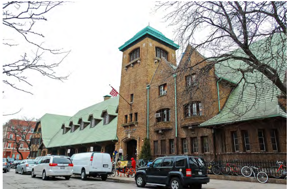
Zimmerman also served as architect to Chicago's West Park Commission from 1907 to 1914, designing a number of fieldhouses and other park facilities, including (bottom) the Pulaski Park Fieldhouse at 1419 W. Blackhawk St. (a designated Chicago Landmark).
