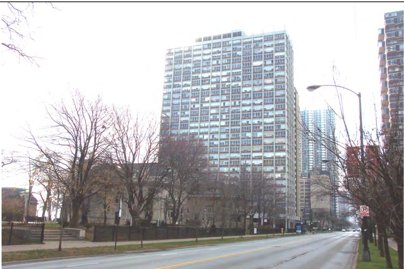
Top: The imminent demolition of the Axel Strom house at 6039 N. Sheridan Rd., and the larger issue of the ongoing demolition of mansions on the street, was the subject of an article in the March 2, 1969, Chicago Tribune . Bottom: A view of North Sheridan Rd. looking south from roughly 6240 North. Berger Park, with its surviving mansions and coach houses, is in the foreground, while apartment towers can be seen in the blocks to the south.
