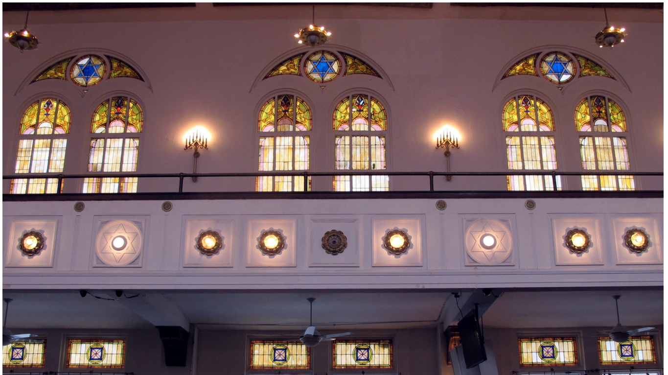
The interior of the former synagogue, now church, includes an unusual cantilevered balcony that eliminates the need for intrusive columns. Though the building became a Christian house of worship in 1954, the congregation has preserved the Torah ark and other Jewish symbols on the interior.
