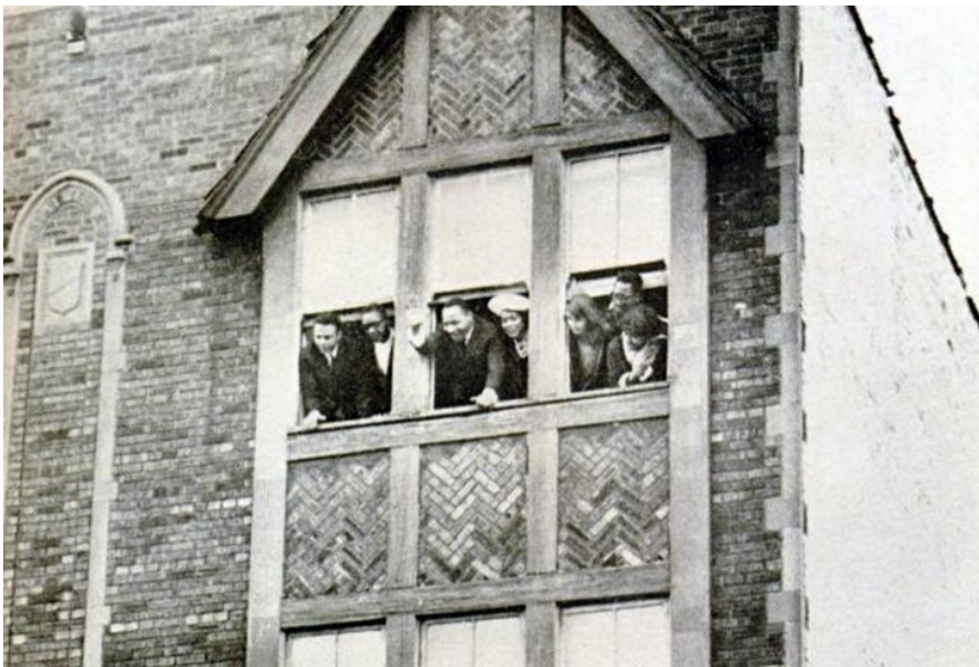
To immerse himself in the problem of the city's slums, King moved into a run-down North Lawndale apartment at 1550 S. Hamlin Avenue (left) which was found by Rev. Stone and located a few blocks from the Stone Temple Baptist Church. ( Ebony , April 1966)
