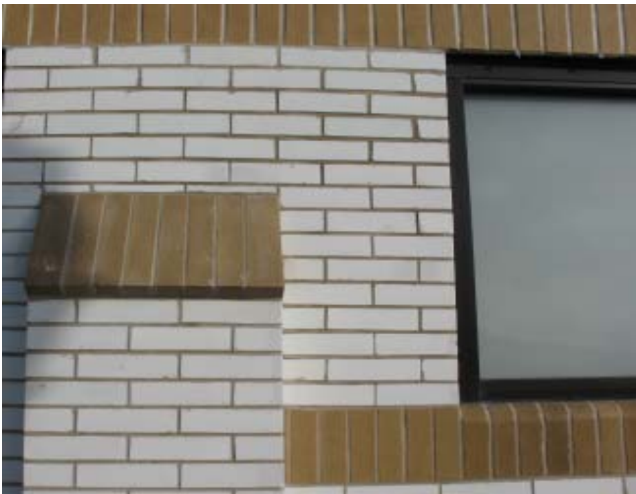
Top: A close-up view of the building's corner tower, with its buttresses and green-brick accents. Bottom: The building's exterior walls are constructed of white-glazed brick with beige-brick detailing that accents windows and copings.
