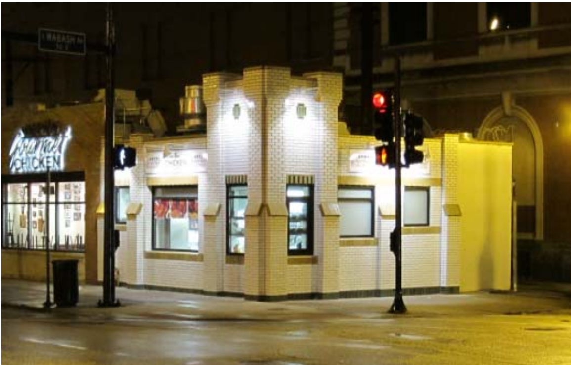
Top: White Castle # 8, located in Minneapolis, is listed on the National Register of Historic Places. It was built in 1936 from a prototype design using porcelain-enamel steel panels.
