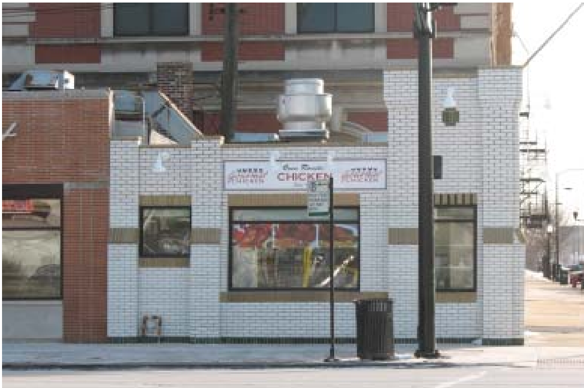
White Castle #16 is a small commercial building built of white-glazed brick with green and beige brick trim. Its corner location, visually-prominent corner tower, and crisp form and detailing give the building a visual scale that belies its diminutive size. The building's design was a standard one used by White Castle in the late 1920s and early 30s.
