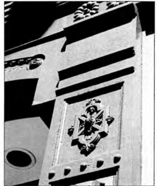
The Halsted Street storefront retains its original 1887 appearance. The ornament surrounding the store entrance includes bold geometric and foliate patterns rendered in cast iron.
