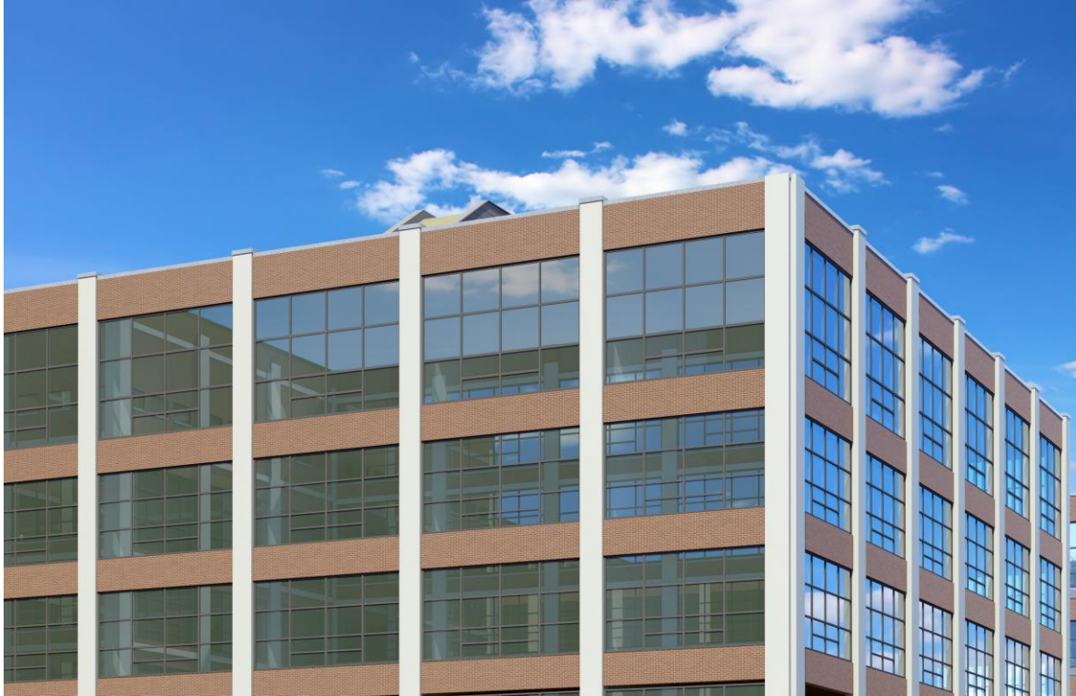
BUILDING B STAIR POP-UP – SW VIEW
