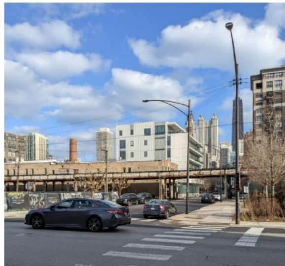
C VIEW LOOKING EAST AT ORLEANS ST & CHESTNUT ST
