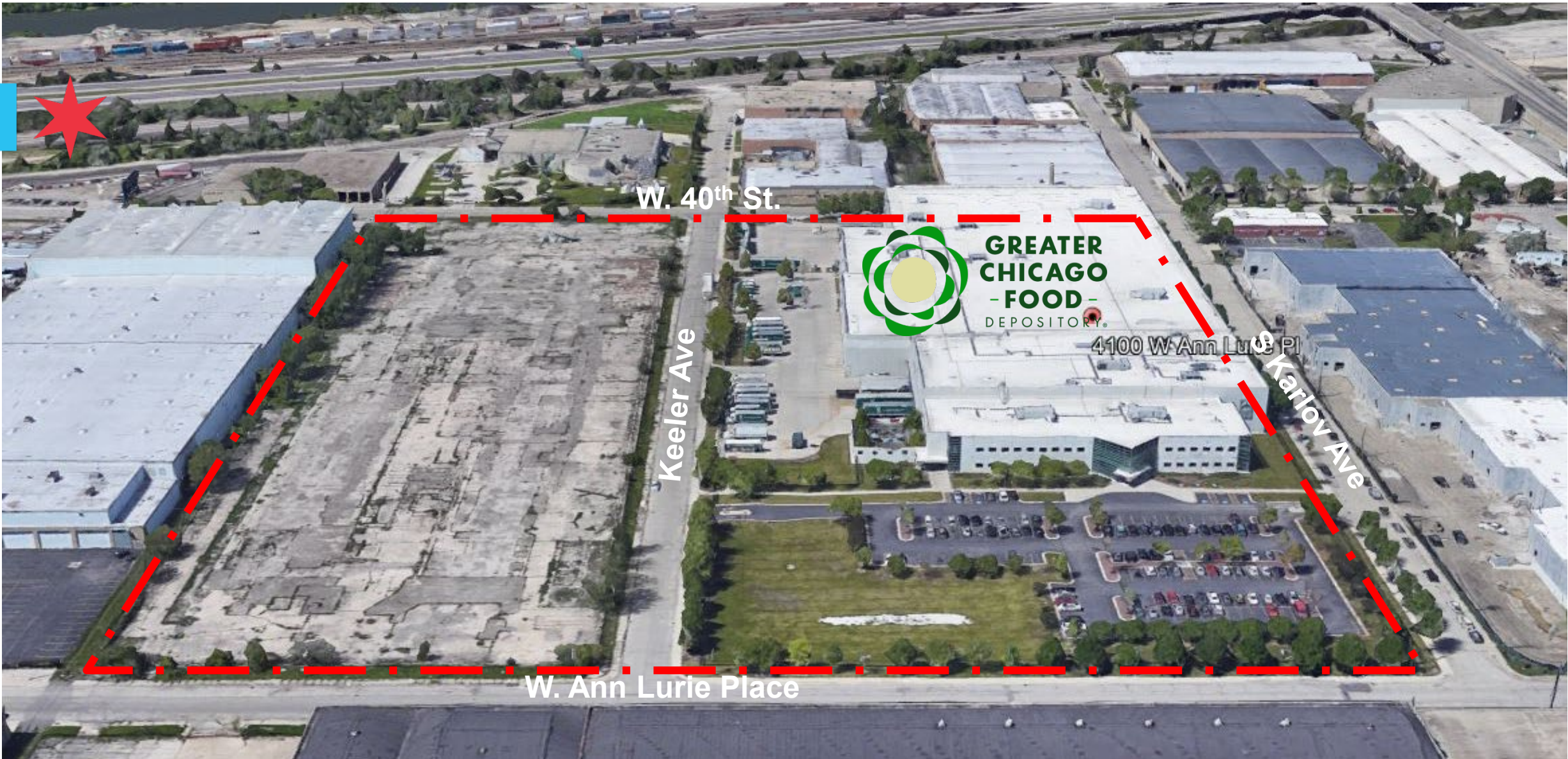
EXISTING SITE AERIAL LOOKING NORTH
