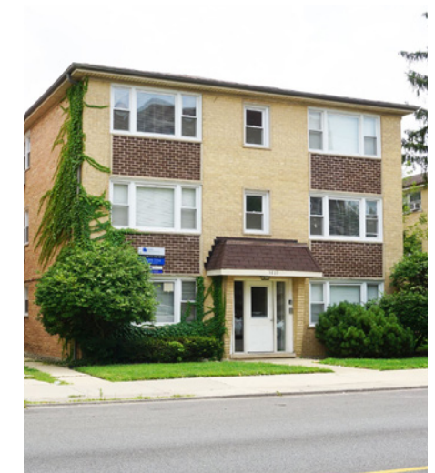
Figure 21. Multi-unit apartment - 3025-27 N Harlem Avenue
