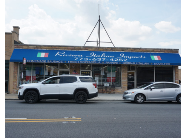
Figure 17. One-part commercial block - 3220 N Harlem Avenue
