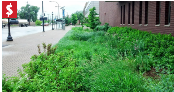
Figure 38. Native plant rain garden along the Cermak/Blue Island Streetscape (Source: CDOT)
