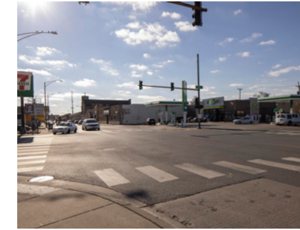
Figure 76. Looking south on Harlem Avenue from Diversey Avenue
