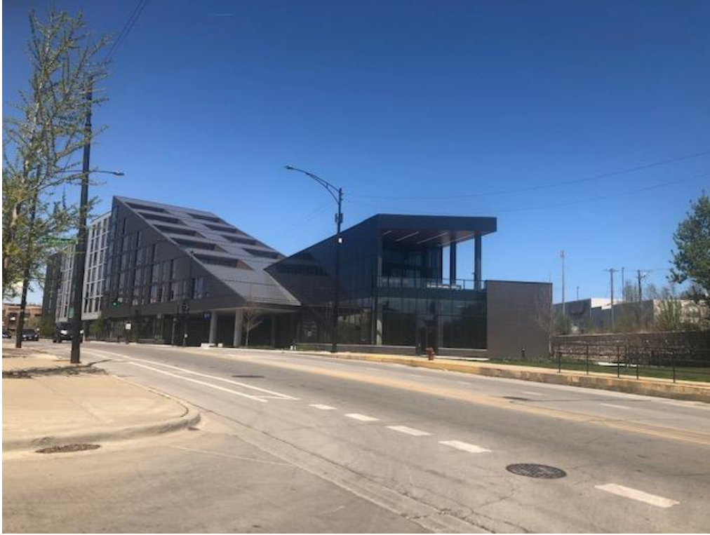
View of PD 1420 Sub-Area A Looking North Along Elston Avenue
