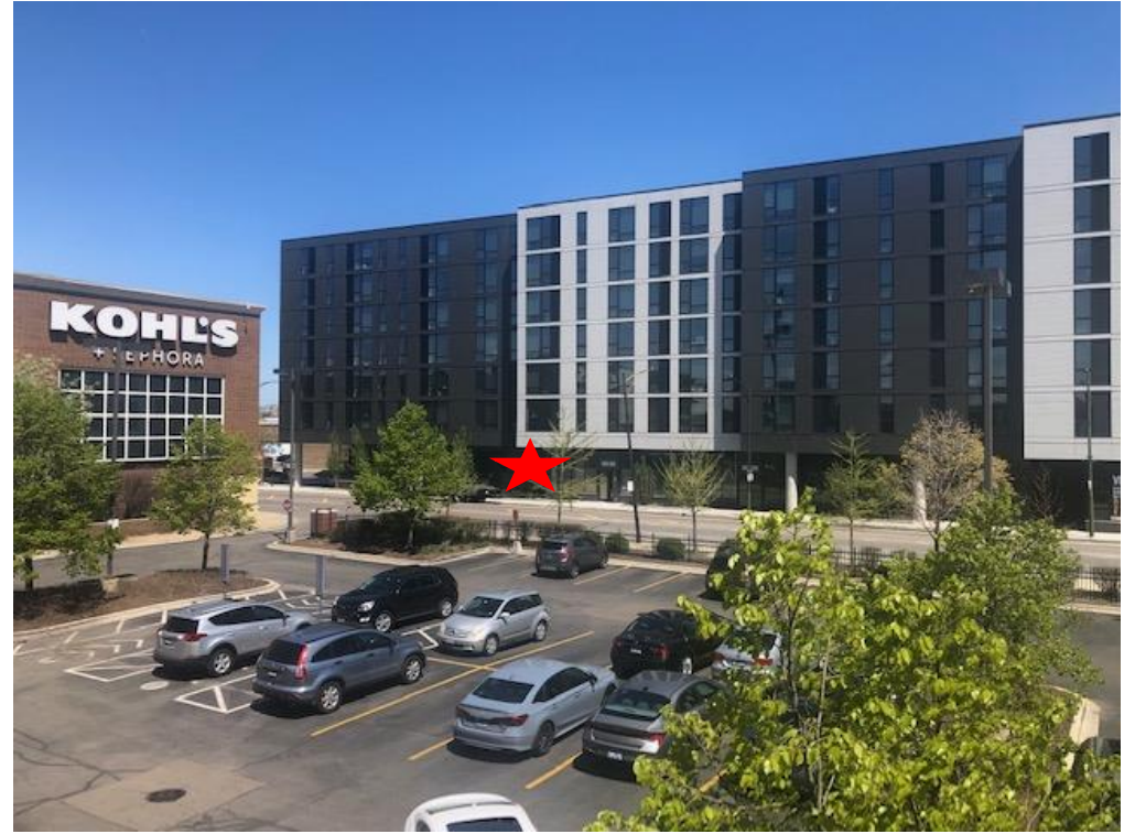
The Proposed New Use will be located on the ground floor of the building approximately where indicated
