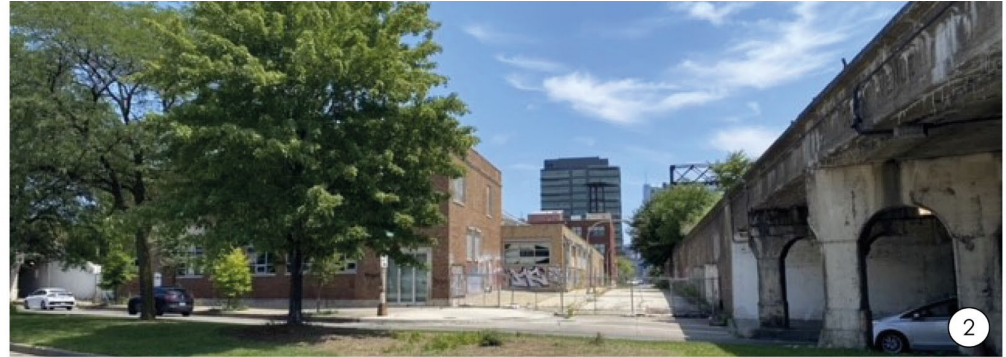
LOOKING SW FROM ELIZABETH ST
