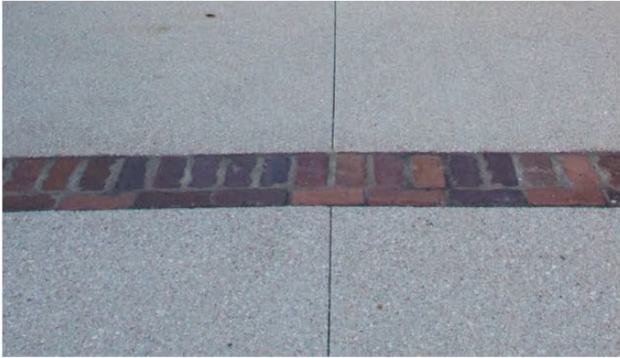
Exposed aggregate pedestrian path with brick accents
