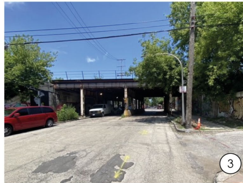
LOOKING SW FROM ELIZABETH ST
