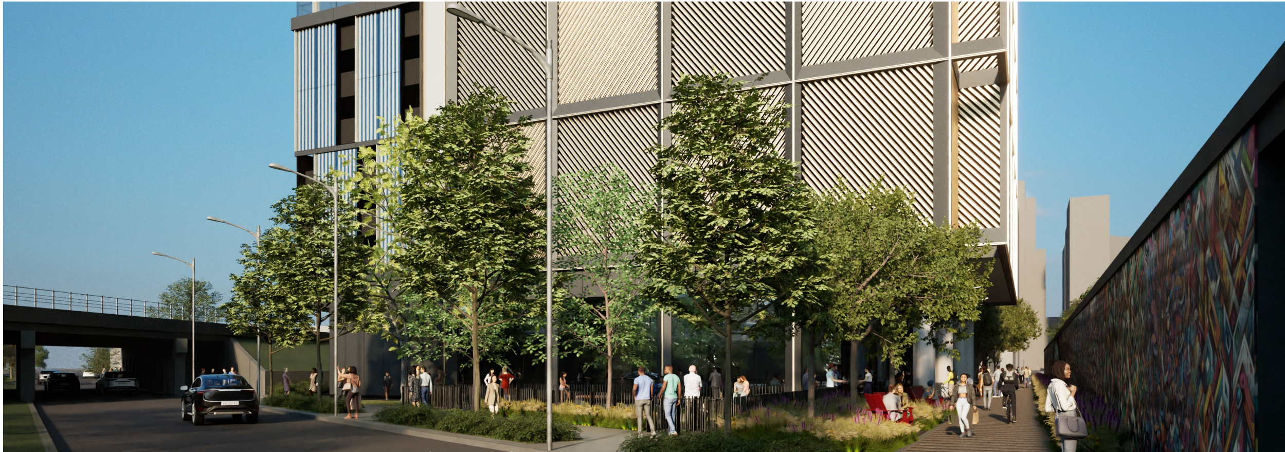
PEDESTRIAN CONTEXT _ View Looking Northeast from N. Odgen Ave. & W. Kinzie Ave.
