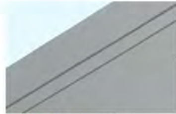
Painted Architectural Concrete W/Reveals
