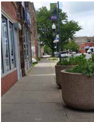
Existing underutilized planters on 75th Street
