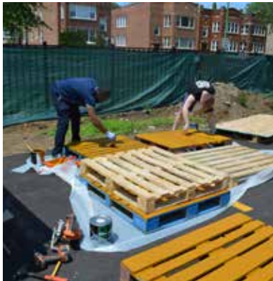
Design team constructing parklets at A&S Beverages
