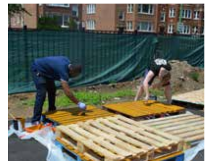
Design team constructing parklets at a local business parking lot
