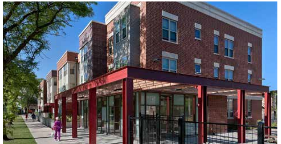
Infill housing development The Jackson at Woodlawn Park - Chicago, IL
