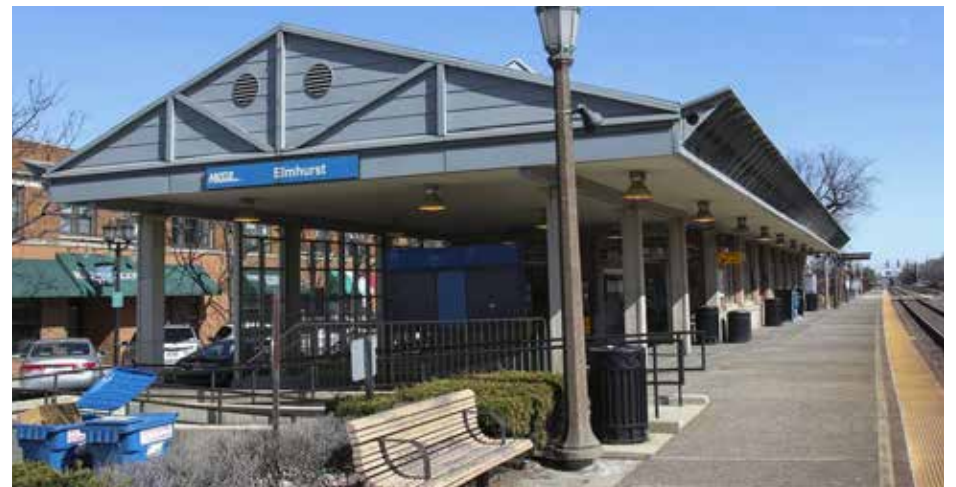
Upgraded Metra Station - Elmhurst, IL
