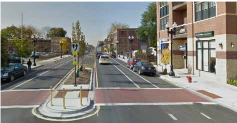
Upgraded pedestrian crossing - Chicago, IL
