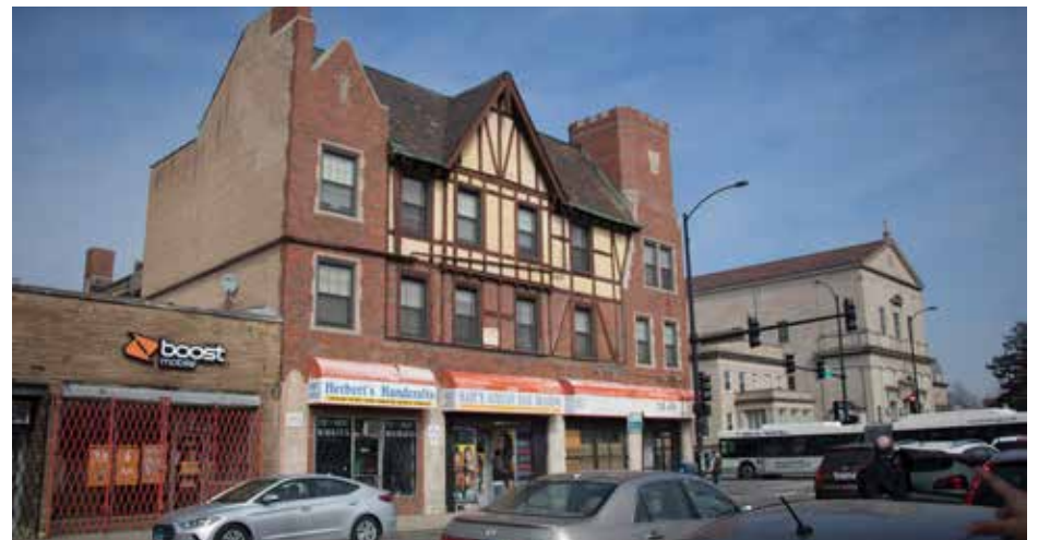
Typical mixed use retail+residential along the corridors
