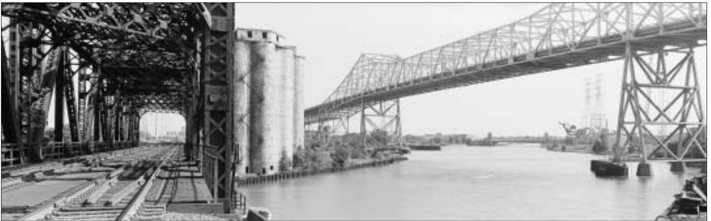
Chicago Skyway and the Waddell and Harrington Lift Bridge over the Calumet River.
