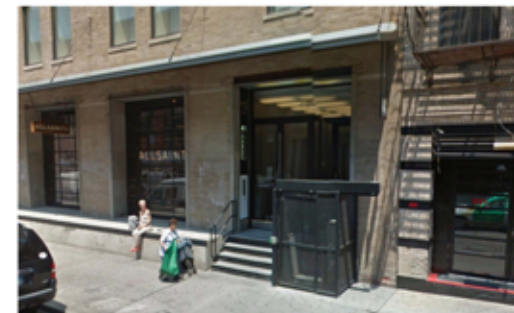
Example of limited railing use. Portions of existing loading docks can be removed to efficiently create ADA accessible entries with steps and elevators
