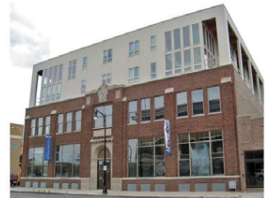
Example of inappropriate rooftop addition. Do not add directly above parapets.
