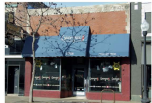
Do not cover ornament or other character defining building features with awnings
