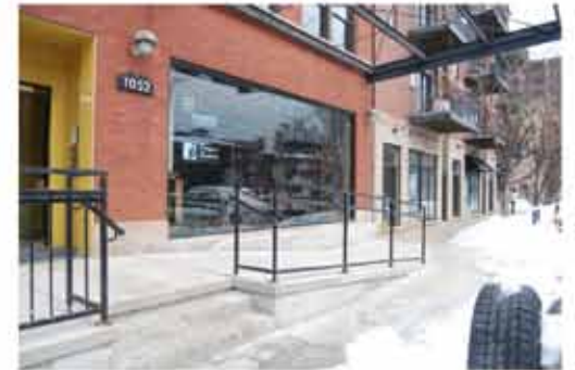
Strong example of creative ADA compliance ramping and railing design along the side street
