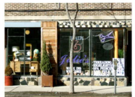
Do not apply cladding over masonry materials
