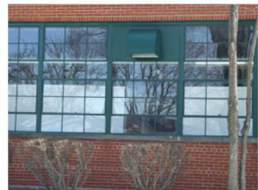
Appropriate new steel windows
