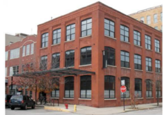
Existing historic canopy frame at Fulton Market
