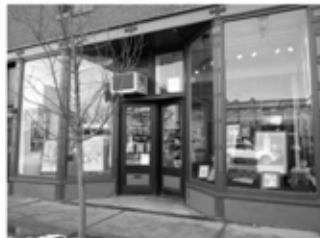
Example of a historic storefront
