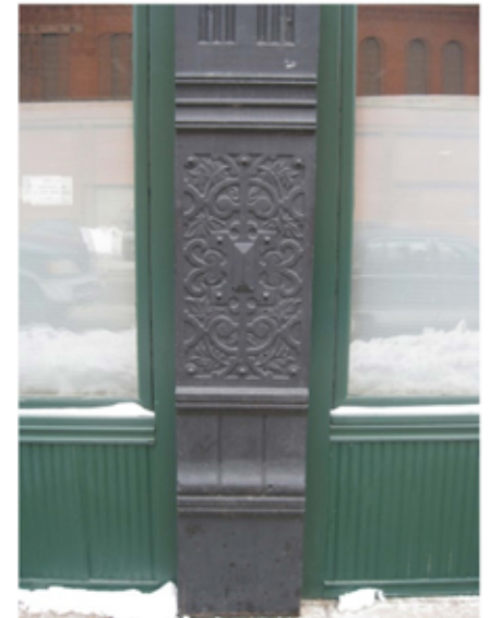
Detail of pier at historic cast iron storefront
