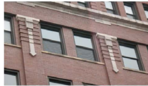
Historic brick masonry with limestone detailing
