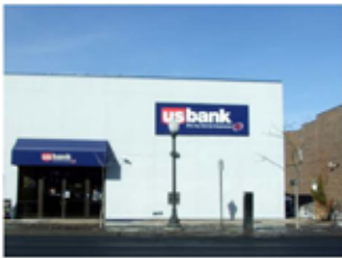
Inappropriate new construction. Blank walls and stucco facades are not compatible with the historic character of the district. Street facades should not be set back from adjacent historic construction.
