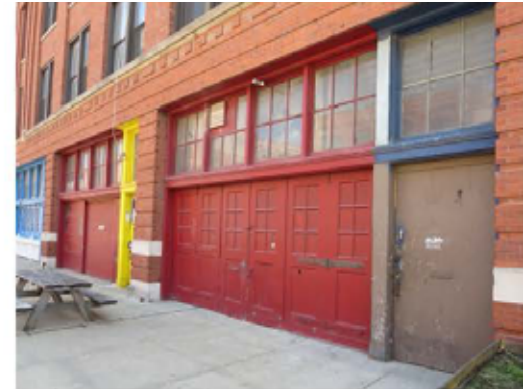
Historic industrial doors at Fulton Market
