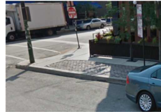
Example of pavers within the parkway
