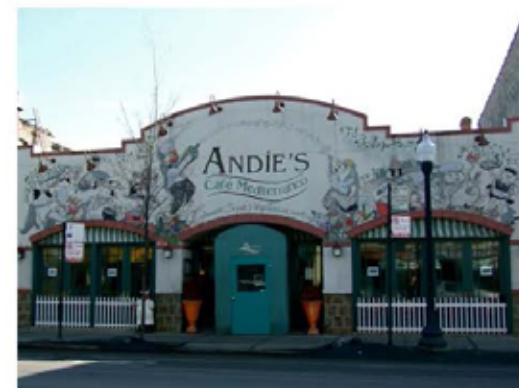
Inappropriate treatment for historic facades - do not cover masonry.
