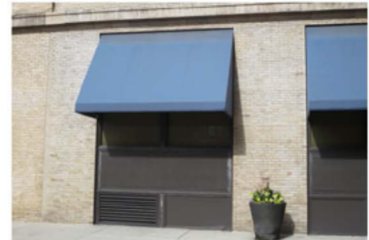
Awnings should be set within masonry openings
