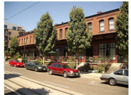
Poor example of landscape use, landscape should not obstruct loading dock use
