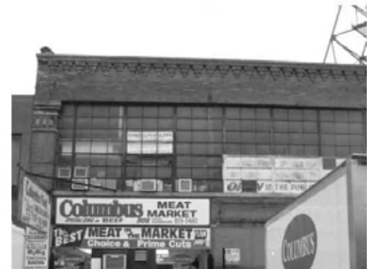
Historic steel windows on Randolph Street
