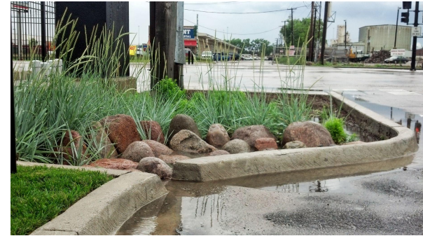
Curb Extension Planter, Chicago
