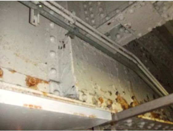
LBP-02: LOWER LEVEL OF MADISON ST. STATION ABOVE STREET.
