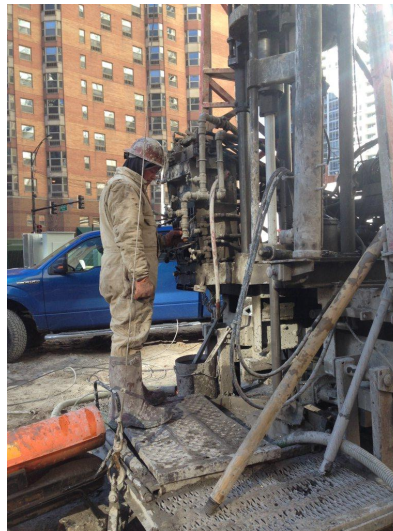
Soil Boring Drilling Rig
