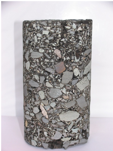
Test Section Pavement Core
