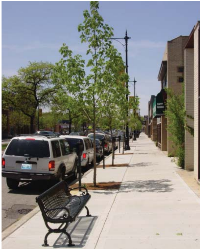
Figure 3-8: 10' width sidewalk condition
