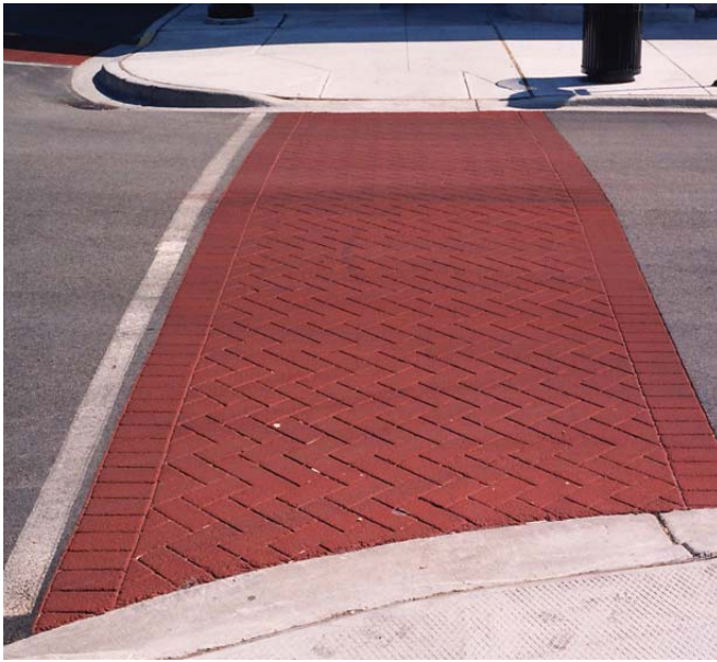
Figure 3-24: Stamped asphalt crosswalk
