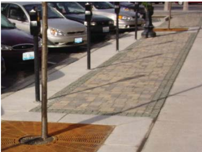
Figure 4-51: Brussels Block unit pavers and tree grates
