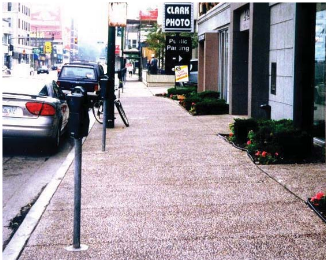
Figure 5-8: Narrow sidewalk condition with flush plantings on private property
