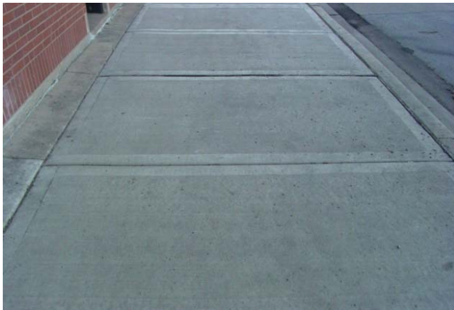
Figure 4-41: Window pane finish concrete
