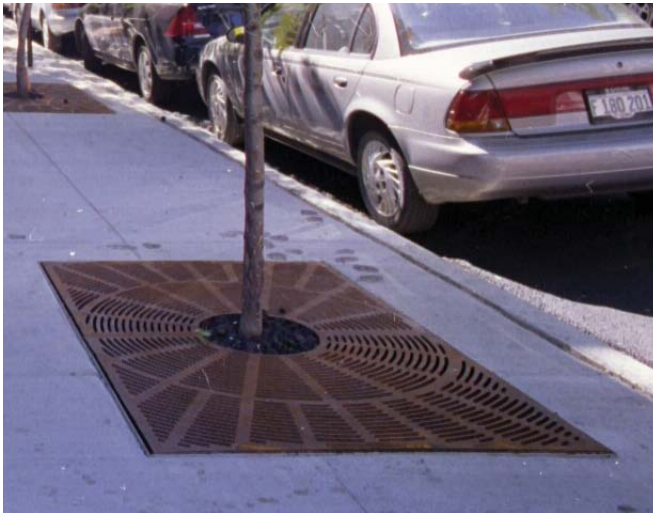
Figure 4-34: Cast iron 4' x 6' tree grate
