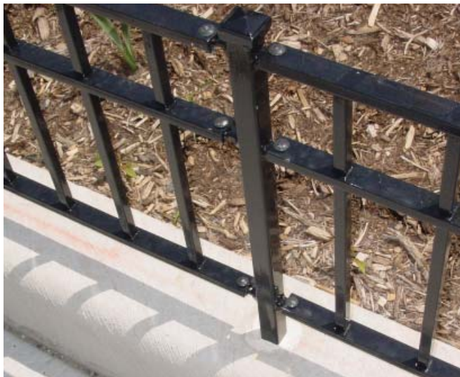
Figure 4-31: Bolted connection of railing panels to post
