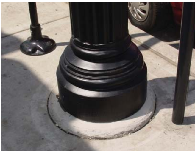
Figure 4-44: Expansion joint at light pole footing
