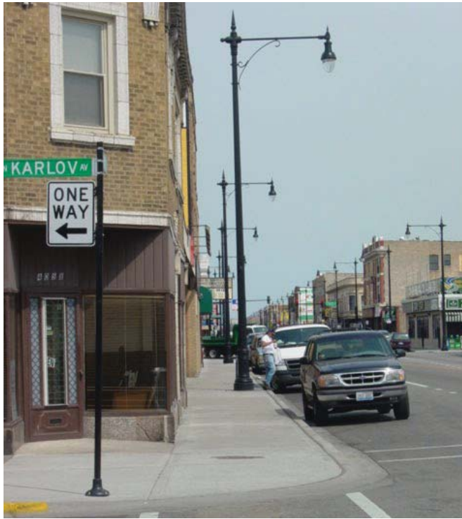
Fig. 5-16: Lawrence Avenue streetscape
