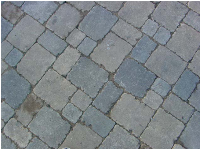
Figure 4-50: Special finish pavers: Brussels Block
