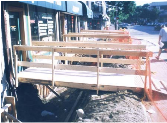
Figure 3-33: Vaulted sidewalk reconstruction
