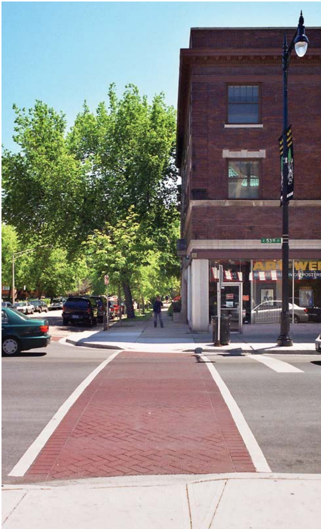
Figure 4-58: Stamped asphalt crosswalk
