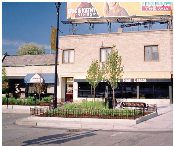
Figure 3-23: Curbed planter at curb extension
