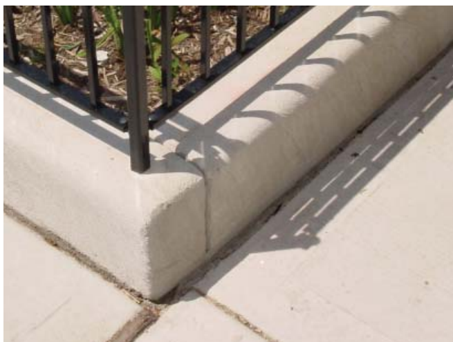
Figure 4-45: Expansion joint at planter curb
