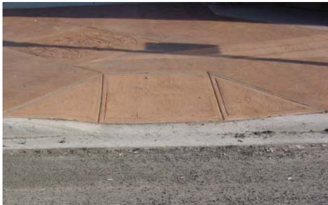
Figure 4-60: Typical curb ramp
