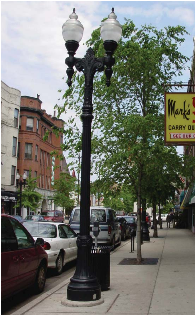
Figure 4-10: Historic Twin Arm pole
