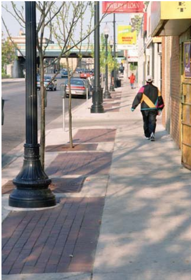
Figure 4-48: Clay unit pavers border this sidewalk
