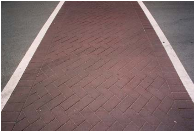
Figure 4-57: Stamped asphalt crosswalk
