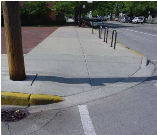
Figure 4-64: Diagonal curbside ramp
