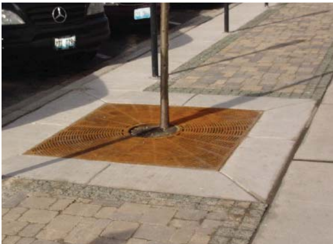
Figure 4-36: 5' x 5' tree grate with concrete band
