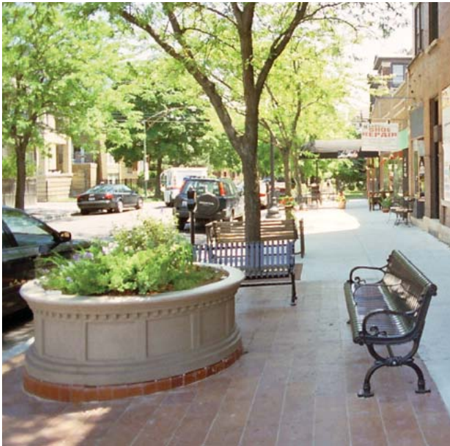
Figure 4-47: Clay unit pavers accent this seating area
