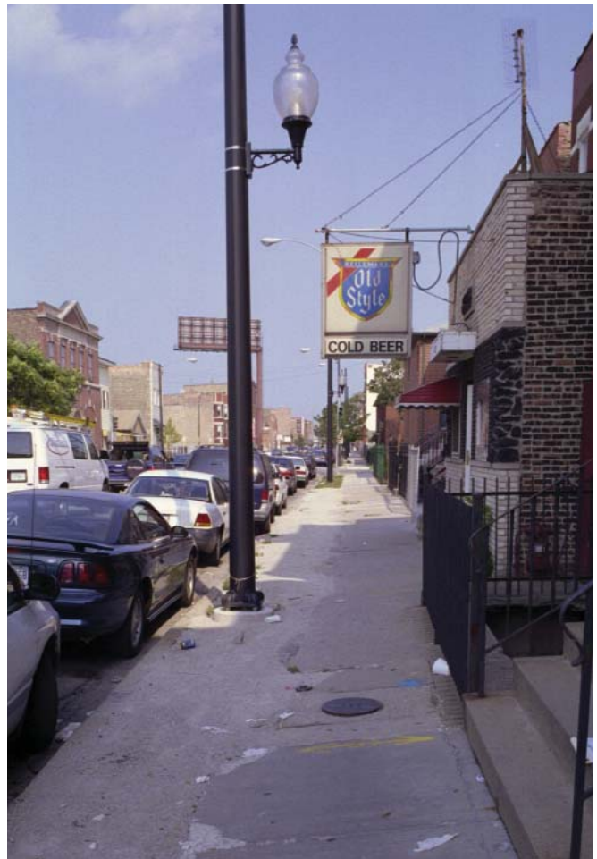
Figure 5-23: Pre-existing conditions for the 26th Street streetscape
