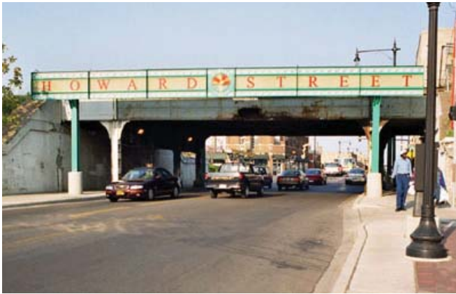
Figure 3-45: Howard Street viaduct
