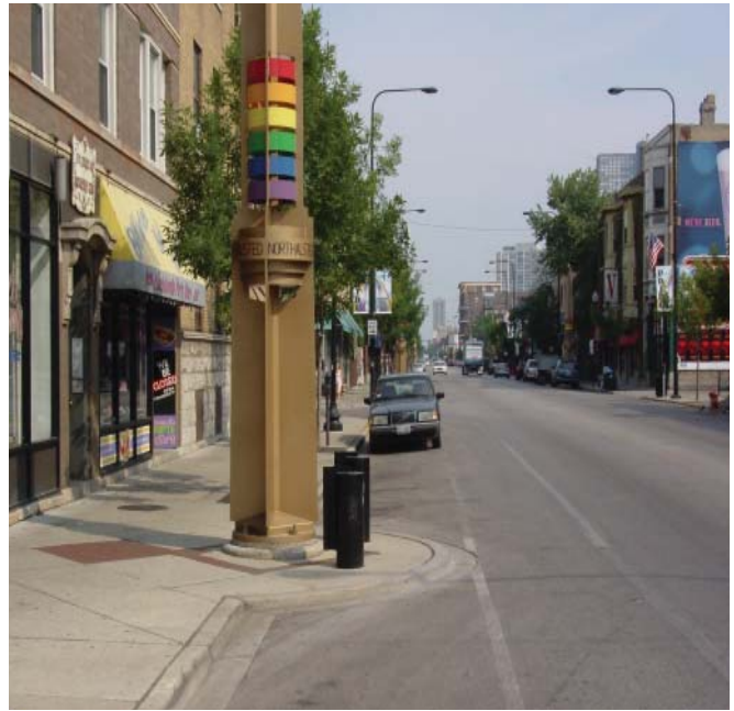
Fig. 5-18: Curb extension allows for placement of community identifier on North Halsted Street
