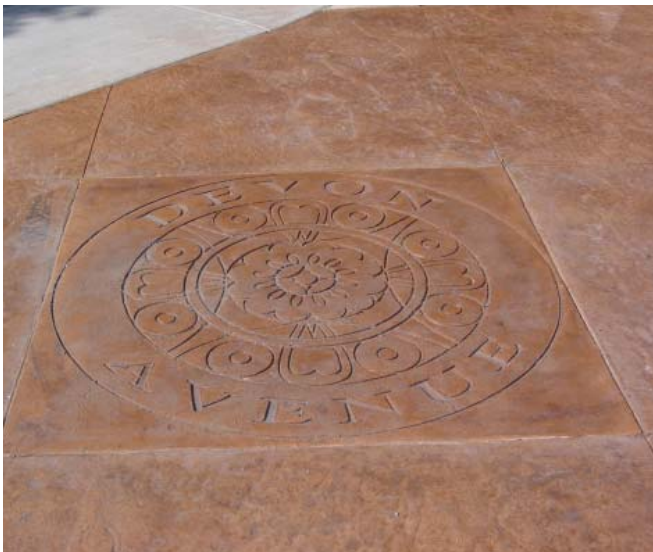
Figure 4-42: Stamped concrete medallion and texture
