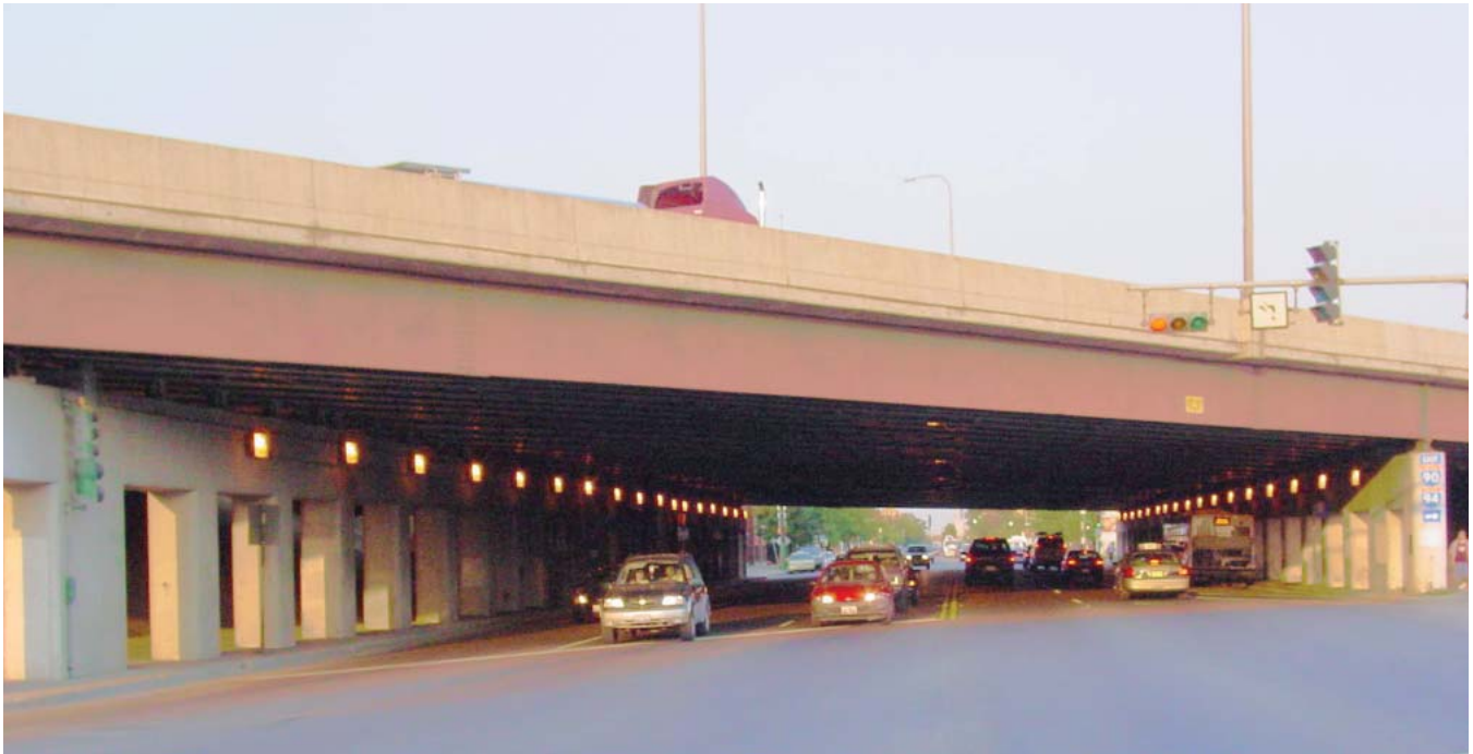
Figure 4-12: Viaduct lighting on Irving Park Road
