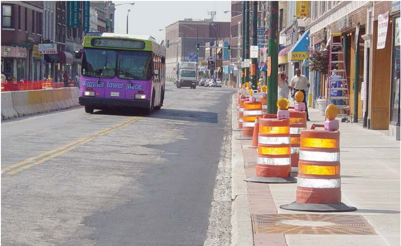
Figure 1-13: During streetscape construction, parking is removed from both sides of the street to allow for uninterrupted two-way traffic flow
