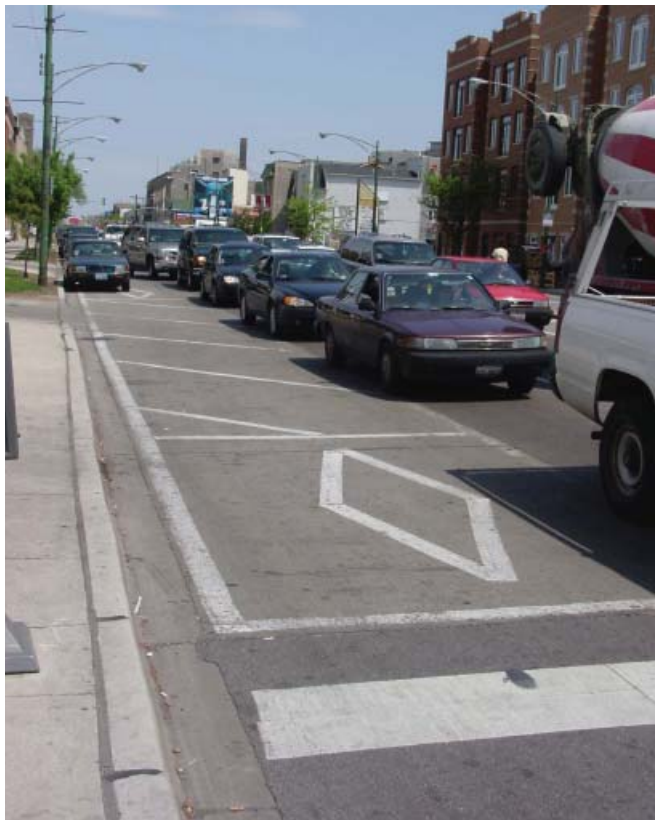
Figure 3-38: Typical bus pad
