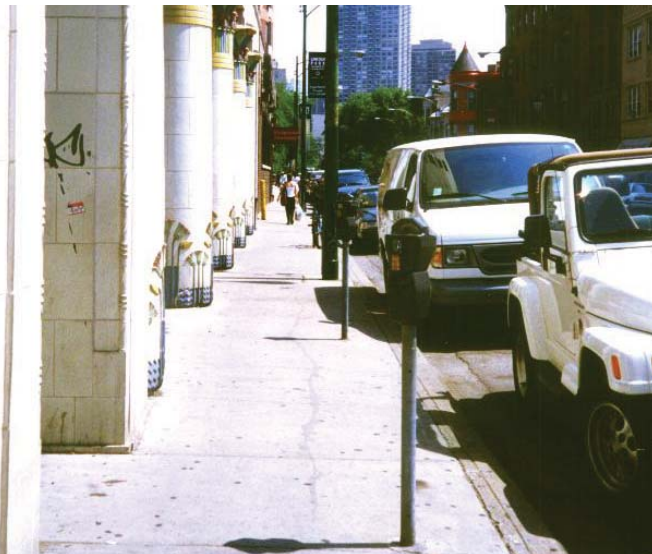
Figure 5-7: Narrow sidewalk condition
