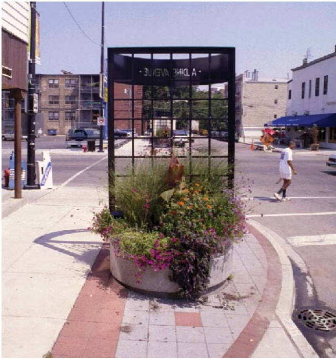
Figure 3-21: Free-standing planter at curb extension
