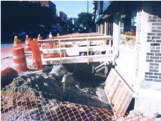
Figure 3-34: Vaulted sidewalk reconstruction
