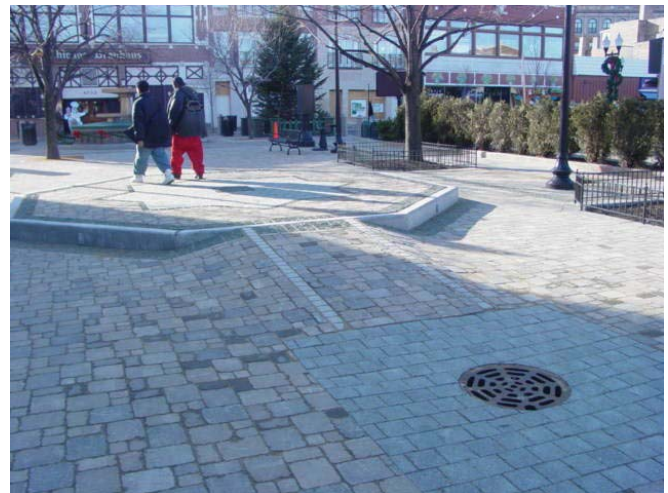
Figure 4-52: Brussels Block unit pavers in Giddings Plaza
