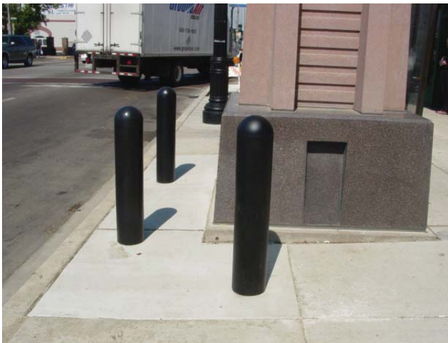
Figure 4-69: Steel pipe bollards
