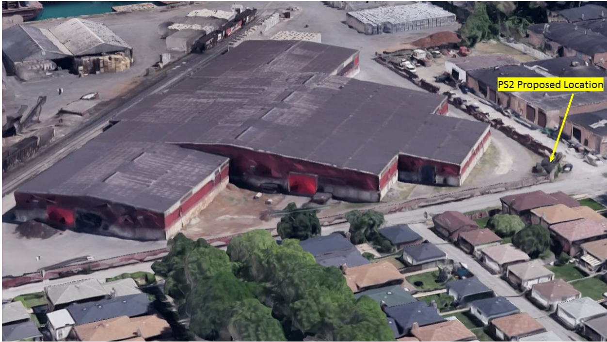
Figure 5 PS2 (Initial Proposed PS2) Site Layout S.H. Bell Facility, 10218 South Avenue O, Chicago, Illinois 60617
