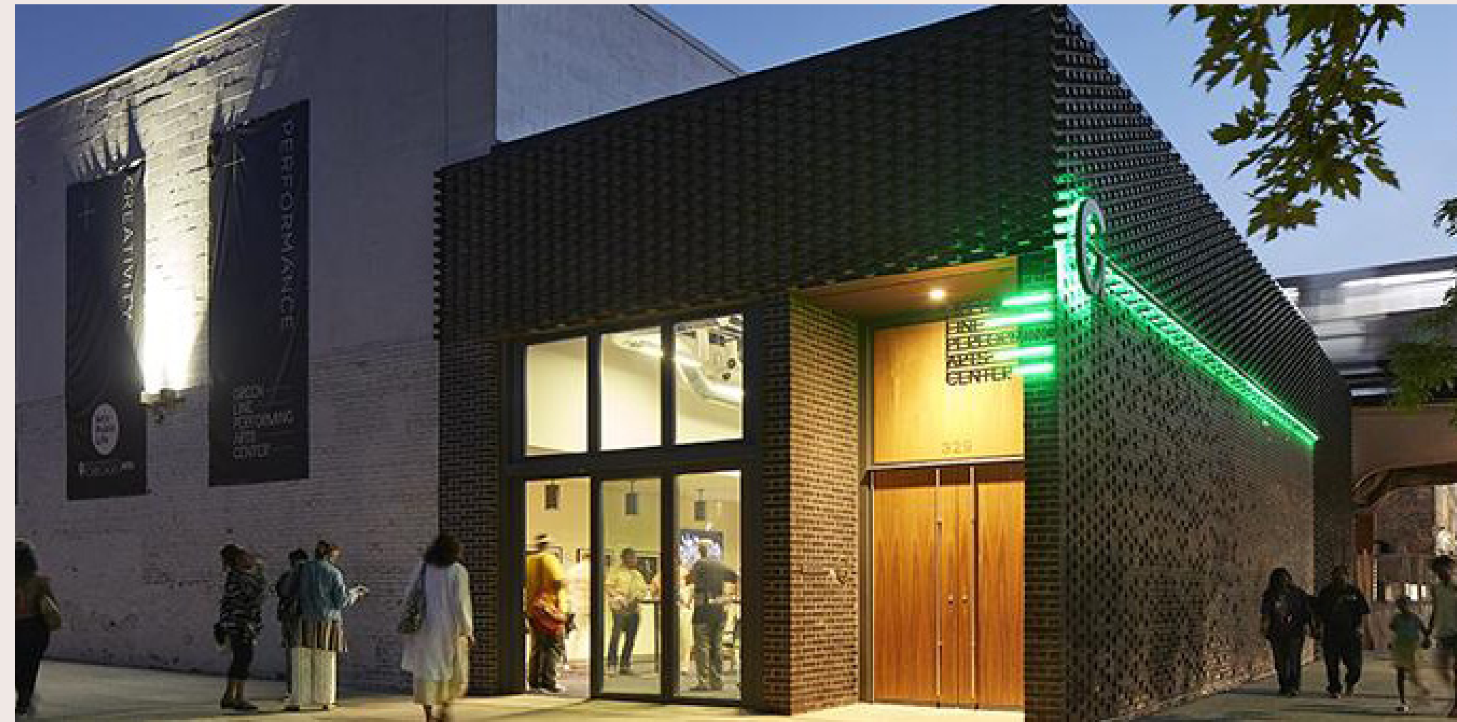
Green Line Performing Arts Center, renovation and addition, Chicago, IL
