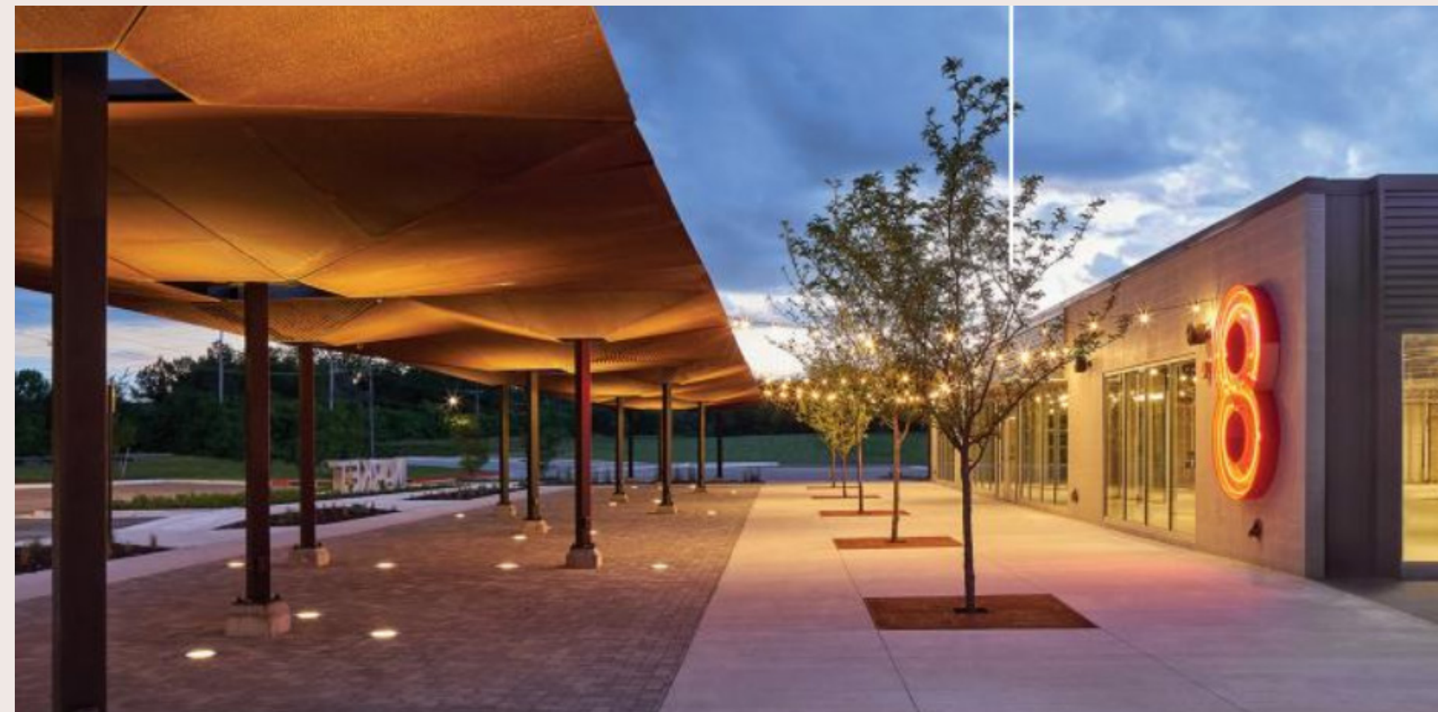
8th Street Market, Bentonville, AK
