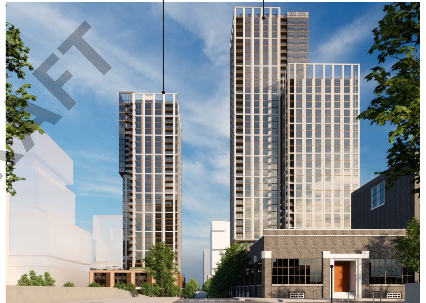
EXISTING MORGAN MANUFACTURING BUILDING
