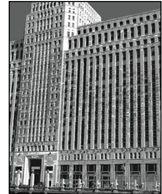
Retrofit Chicago Best Practices Report
