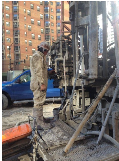
Soil Boring Drilling Rig
