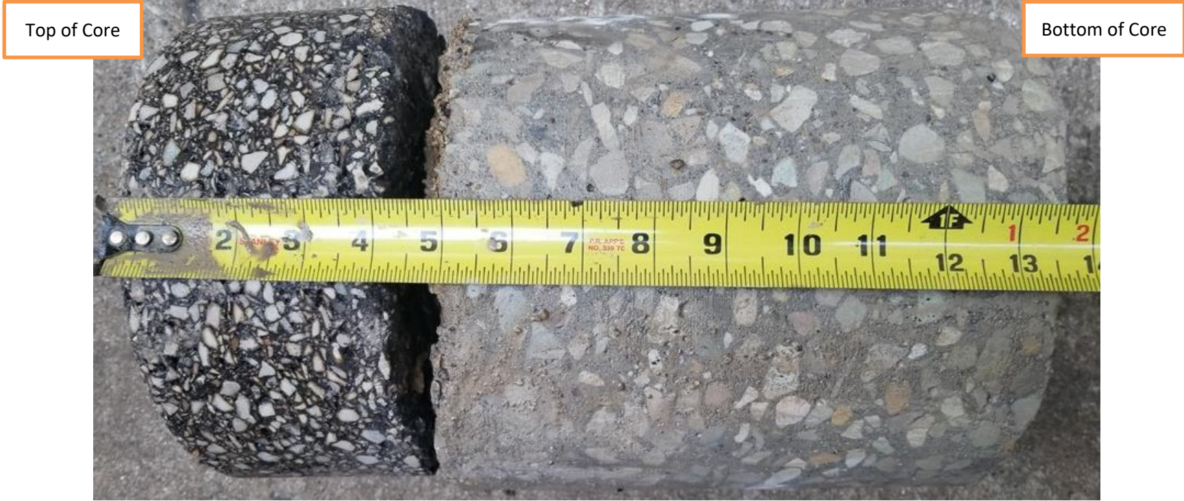
B-04 –Pavement Core
