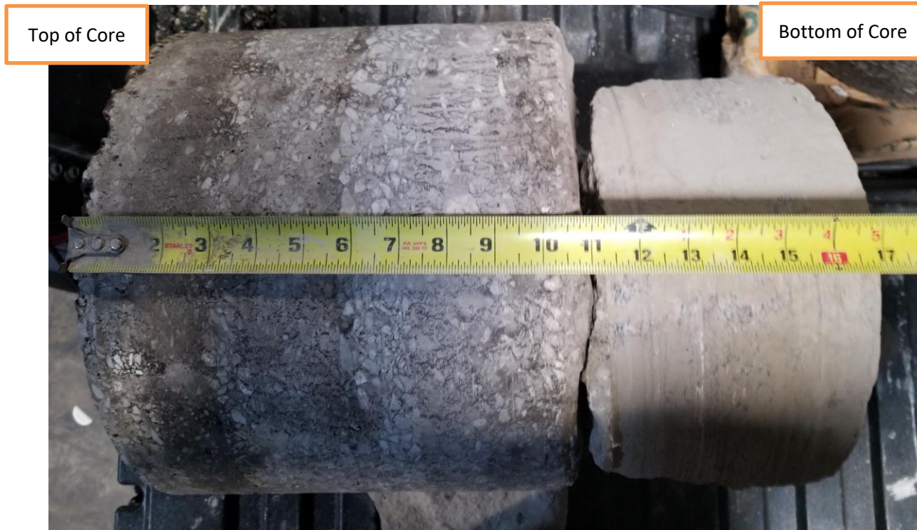
B-08 –Pavement Core
