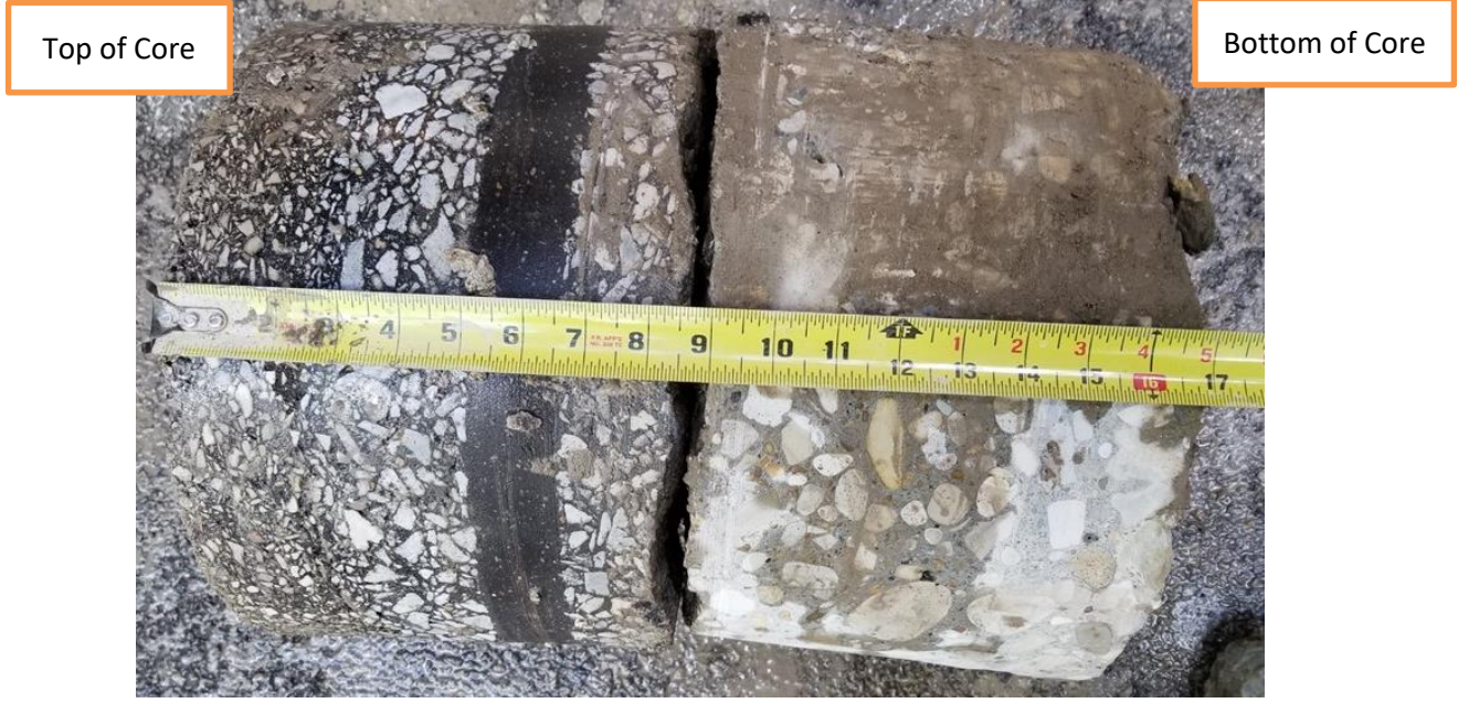
B-05 –Pavement Core
