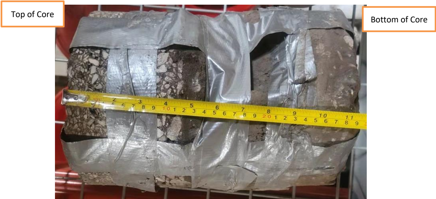
B-03 –Pavement Core
