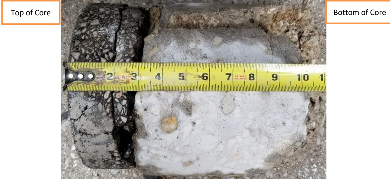
B-02 –Pavement Core
