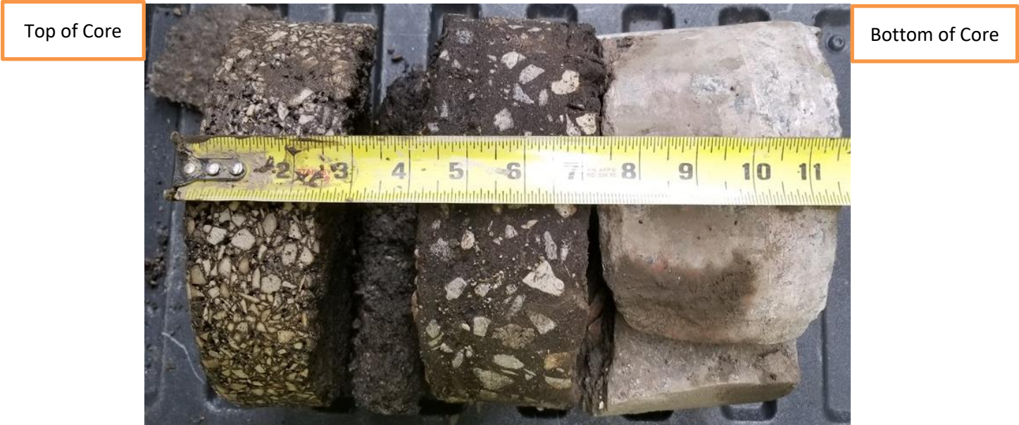
B-01 –Pavement Core
