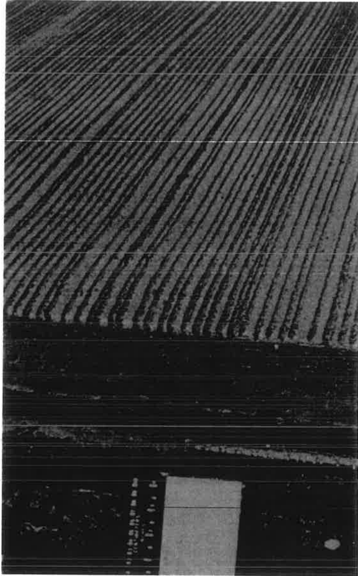
FIGURE 2-5. WIRE COMB TECHNIQUE CONSTRUCTED AT PATRICK HENRY AIRPORT, VIRGINIA, USING A 1/8 INCH X 1/8 INCH X 1/2 INCH CONFIGURATION
