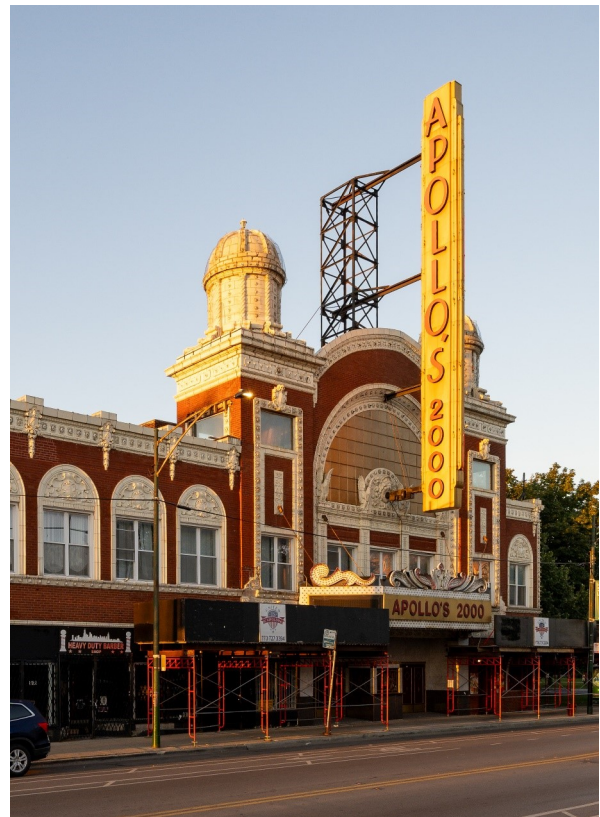
A current photo showing the marquee reduced in width with ornamental flourishes added, and the blade sign refaced.
