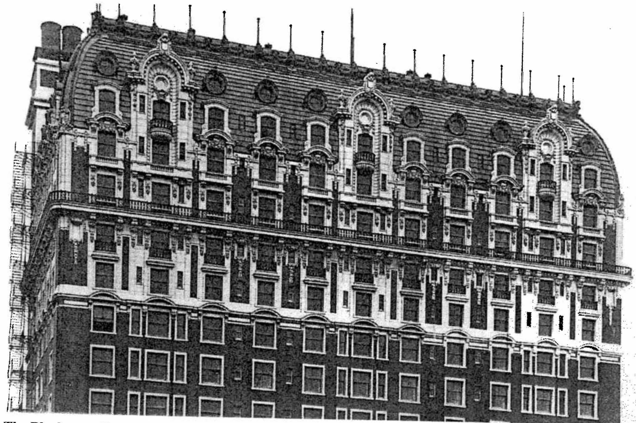
The Blackstone Hotel's mansard roof is one of the most exuberant building tops in Chicago. Several of its original features, however, as seen in this c.1920 photograph (above), are now missing, including a wraparound balcony, decorative roof cresting, ornamental light standards, huge flagpoles (see cover photo), and several terra cotta details (below).
