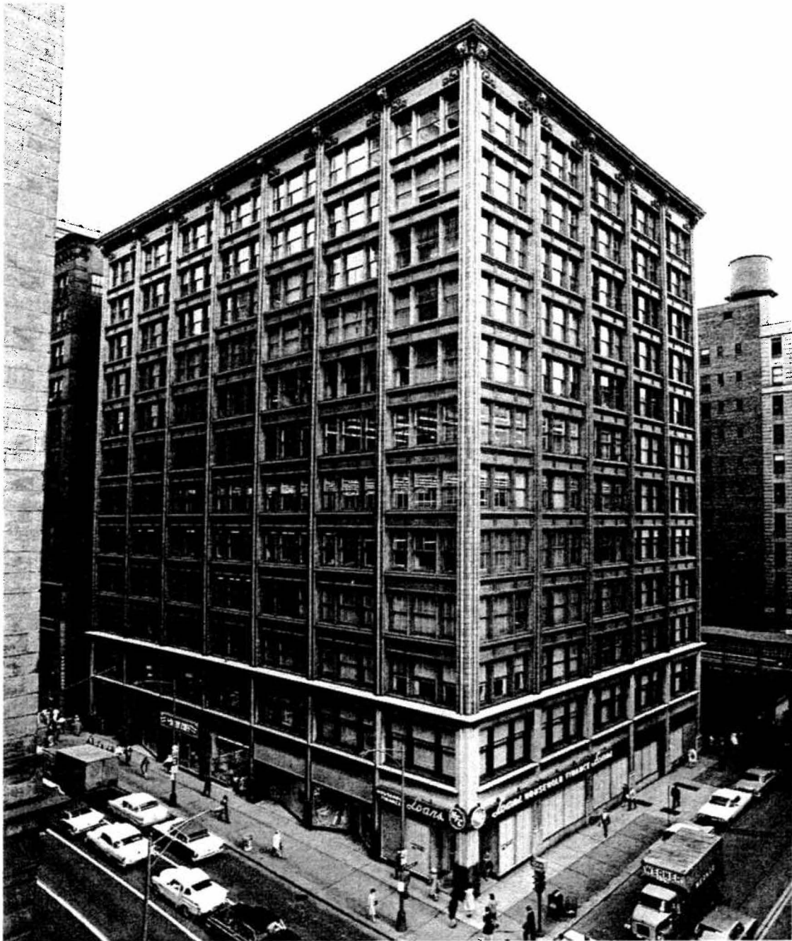
This Richard Nickel photograph of the Brooks Building dates from the 1960s. The building is little changed from its original appearance (see photo on inside front cover), retaining both its original cornice and much of the character of its lower two floors, which are clad in marble.
