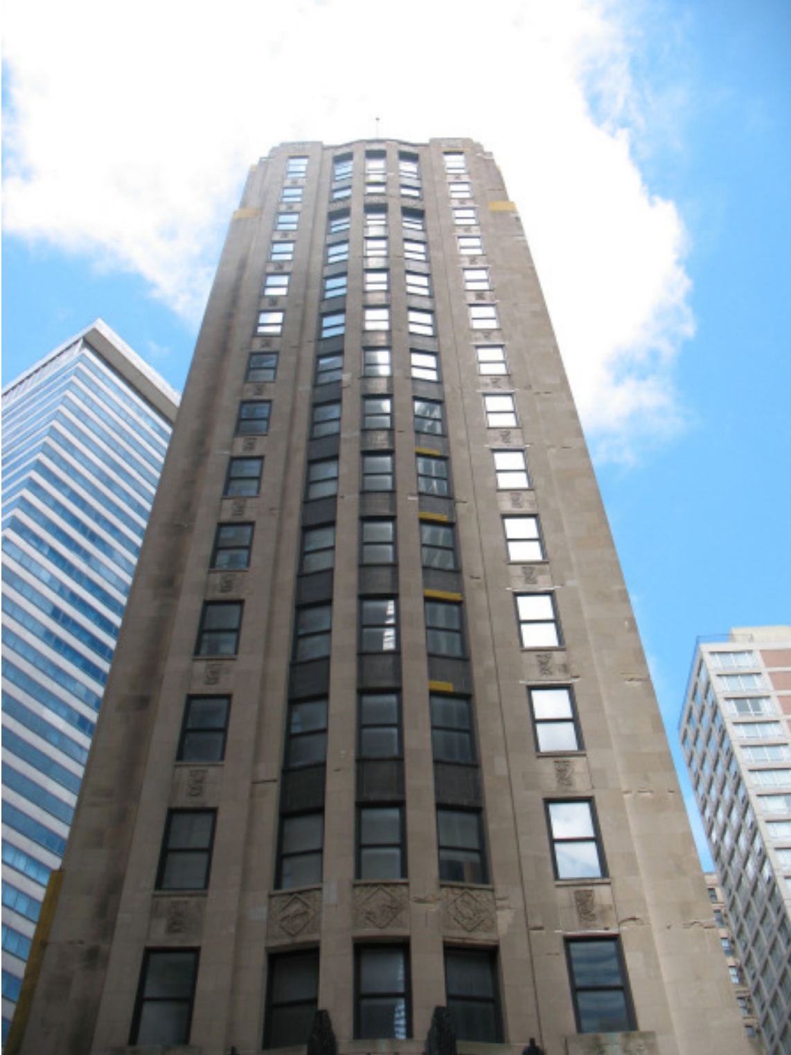
The Chicago Motor Club Building exhibits fine craftsmanship and detailing in materials, including gray limestone, granite and cast-metal.
