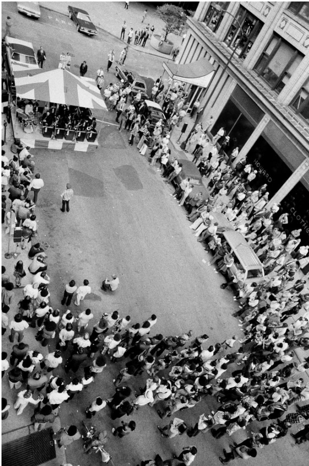
Looking west along Quincy, June 22, 1973. The south elevation of the Consumers Building is at the right side of this photo. Pedestrians gather on Quincy Street, no longer a through-street, for a Friday jazz concert put on by the State Street Council. Terra-cotta piers visible between storefronts have since been covered or removed.
