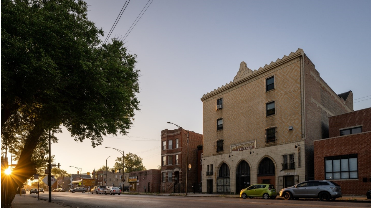
The base of the building is a terra cotta arcade. The large wall expanse and small windows on the upper floors are typical of this building type.
