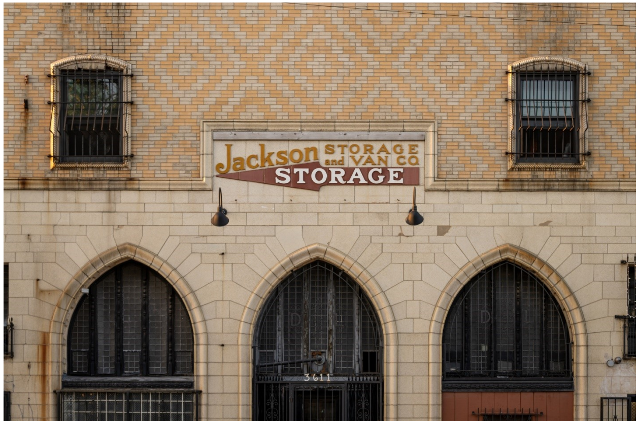
The Jackson Storage and Van Co's logo is rendered in a terra cotta tablet. Light-colored brick set in a tapestry pattern relieves the large expanse of masonry wall on the upper floors.
